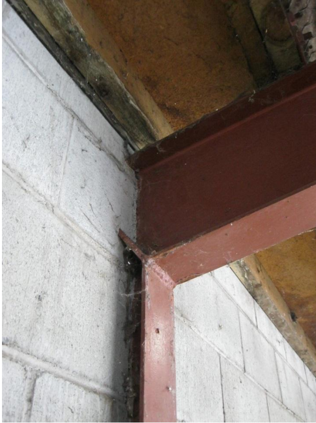
Photograph 11 A typical connection between the steel frame columns and concrete masonry unit walls.
