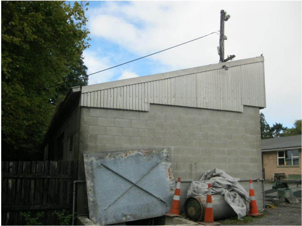
Photograph 3 Western wall of the original pre-1969 pump house attached to the Office Store.
