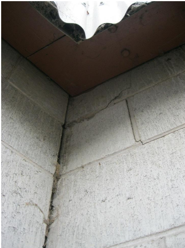
Photograph 6 Cracking to masonry walls at connection between Wings A and B.
