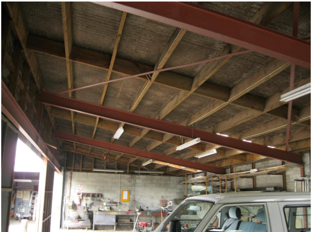
Photograph 10 Roofing system of the Garage portion of Wing B showing timber roof purlins on steel portal frames. Flat steel cross bracing straps are clearly visible.
