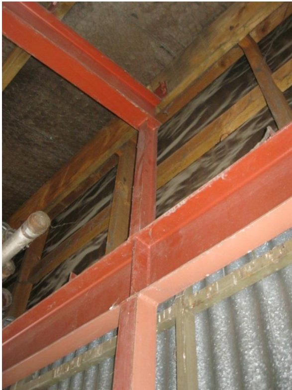
Photograph 12 Typical connections at the western end of the portal frames showing steel beams welded to steel columns.
