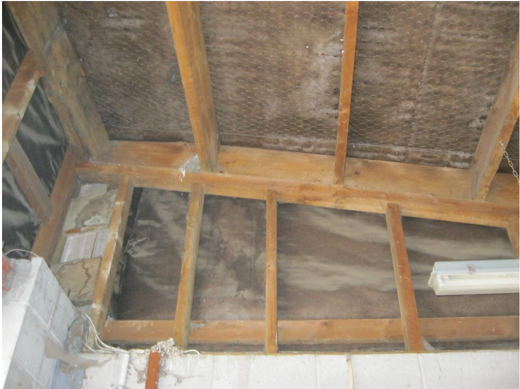
Photograph 9 Timber framed roof supports at the northern end of Wing B.
