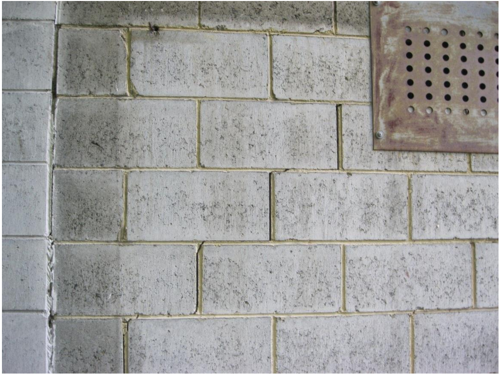
Photograph 5 Cracking to masonry wall of the pre-1969 pump house.
