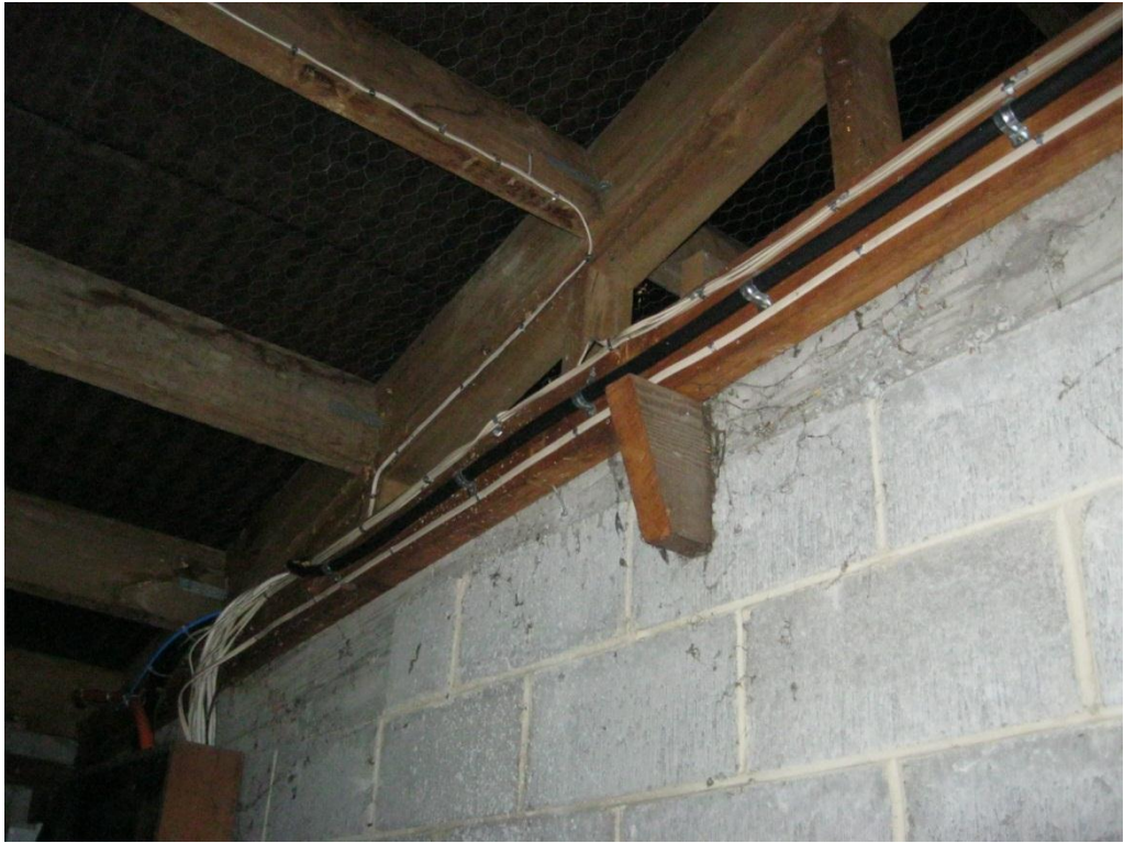
Photograph 13 Typical timber framed roof supports above concrete masonry partition walls.
