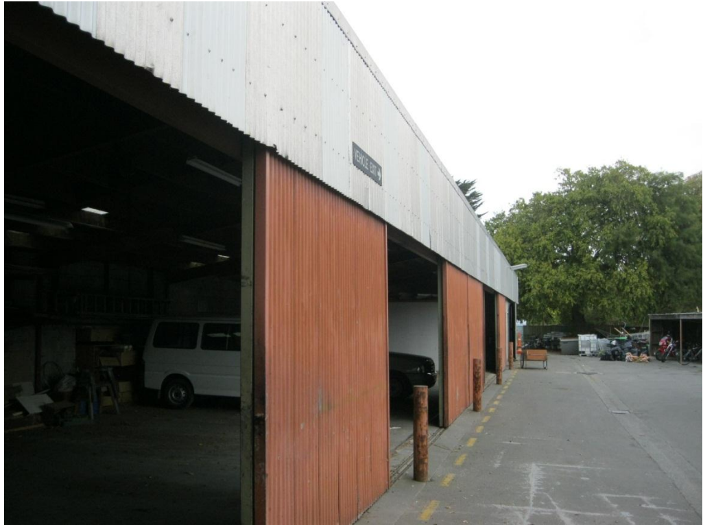
Photograph 7 Western side of Wing B showing the large openings for the garage doors.
