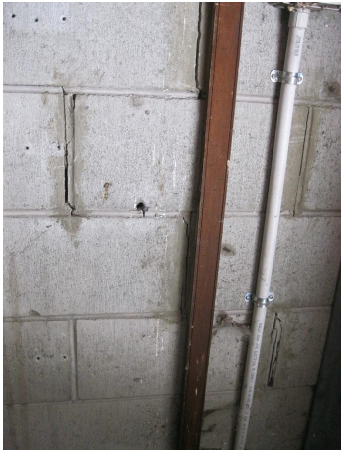
Photograph 8 Cracking to masonry wall at the northern end of Wing B.
