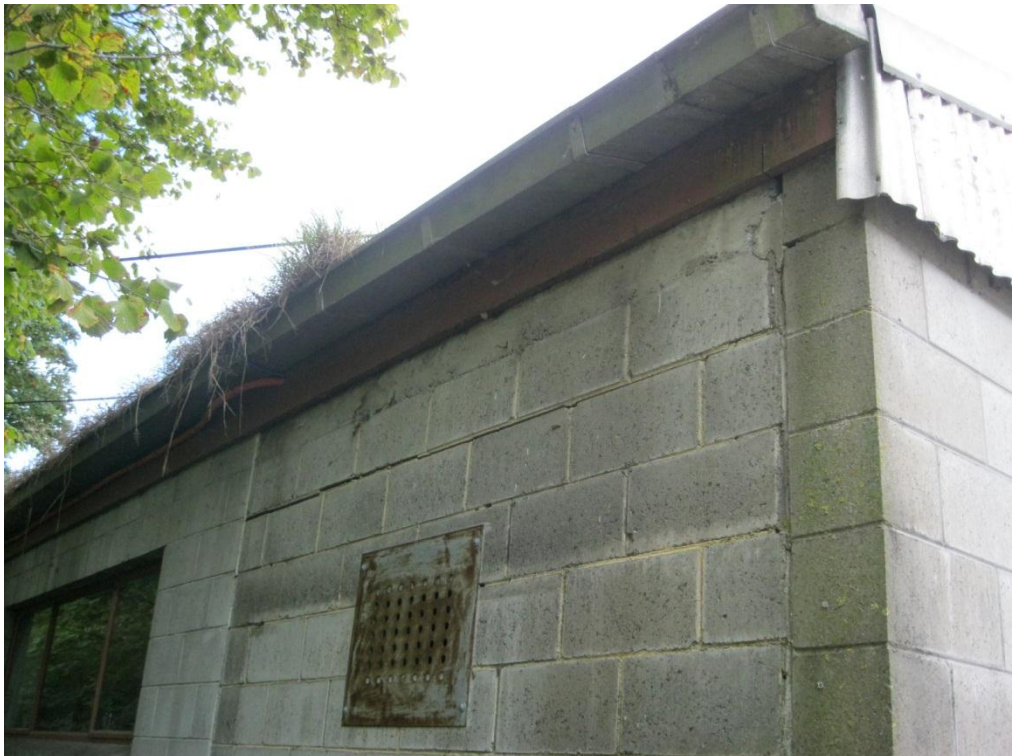
Photograph 4 Connection between pre-1969 pump house and office store building. Horizontal cracking along mortar line is visible.
