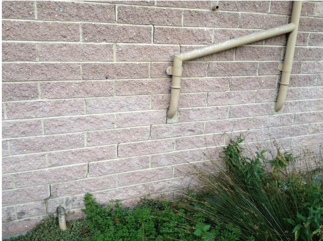
Photograph 5: Shear cracking to brickwork veneer located on south-east of the structure
