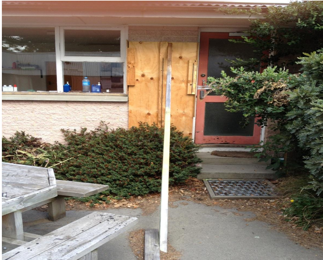
Photograph 7: Temporary propping to brickwork veneer on the north side of structure
