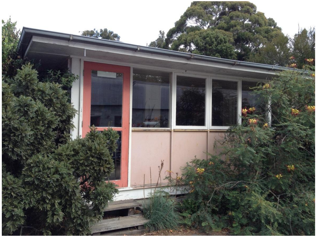
Photograph 3: Flat roof extension to the north side of the structure
