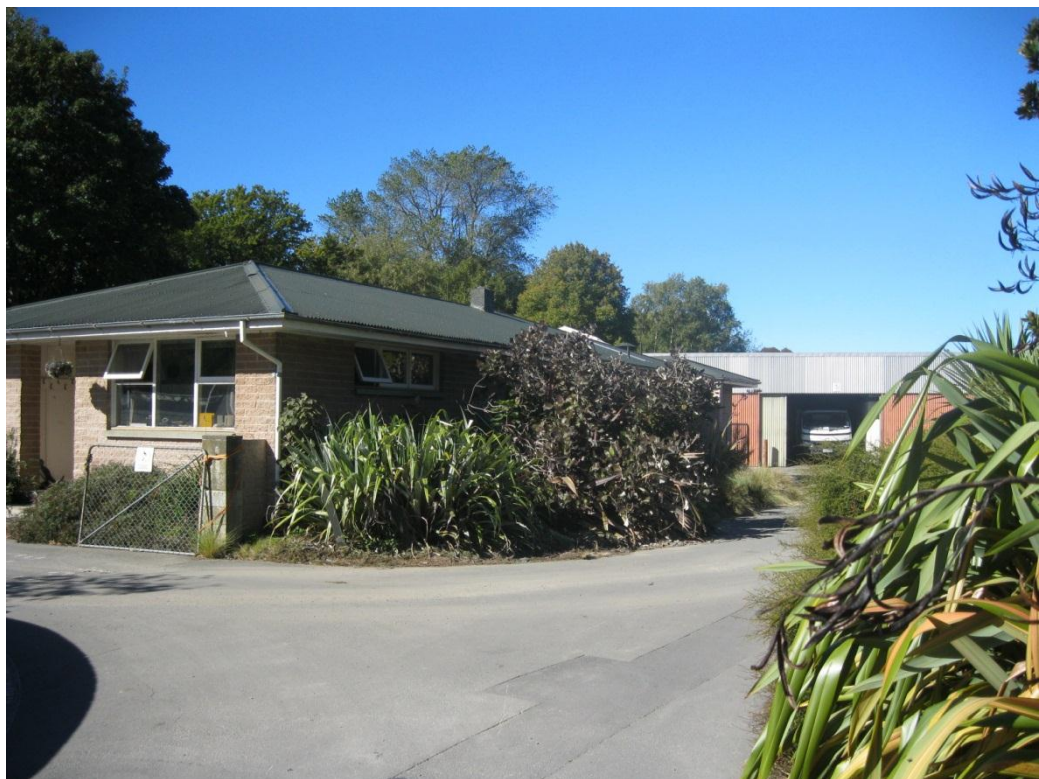
Photograph 2: South and west facing elevations
