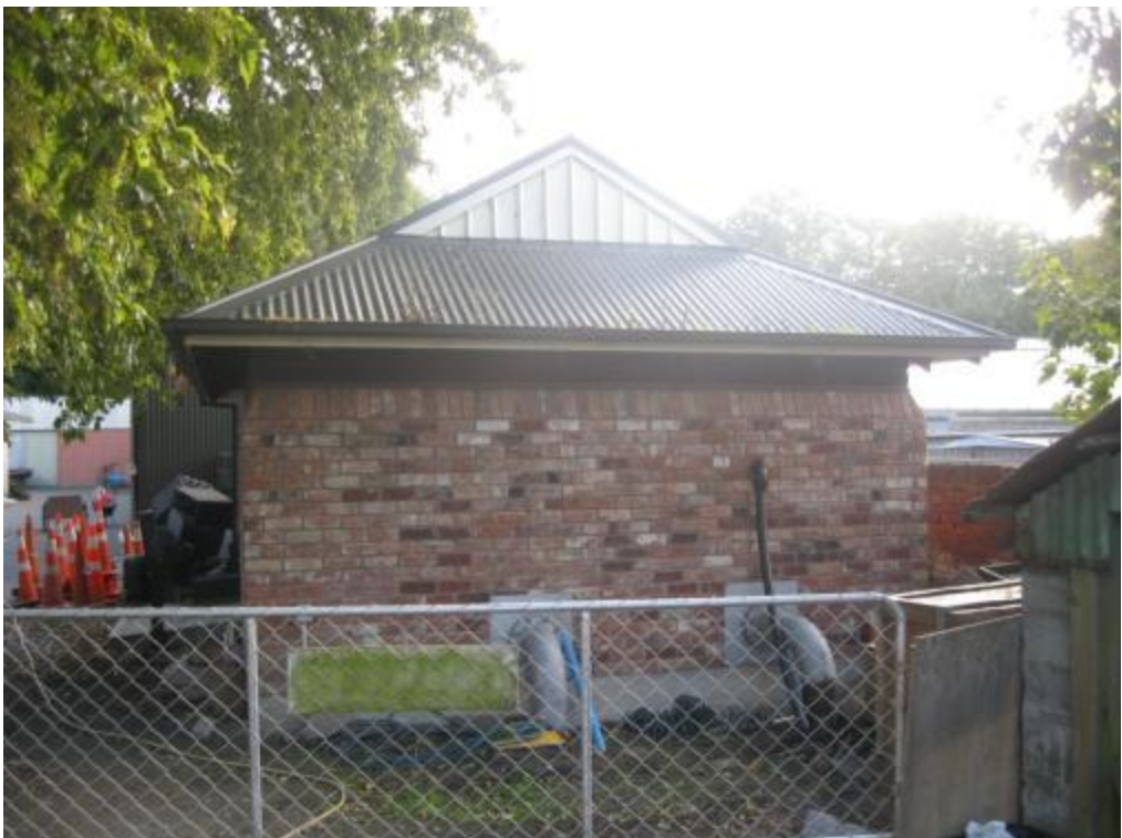
Photograph 2: South facing elevation showing Dutch hip roof
