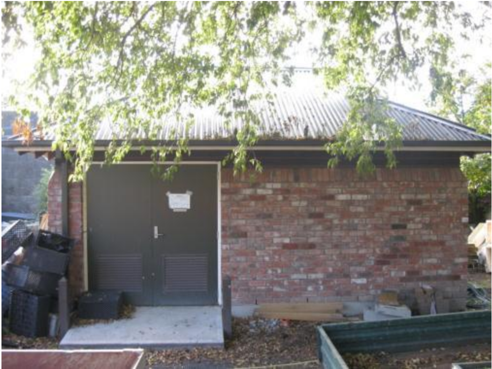
Photograph 1: West facing elevation
