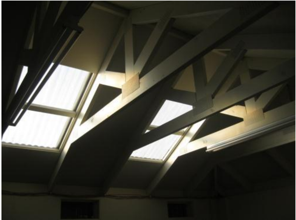
Photograph 3: Skylights to Roof structure
