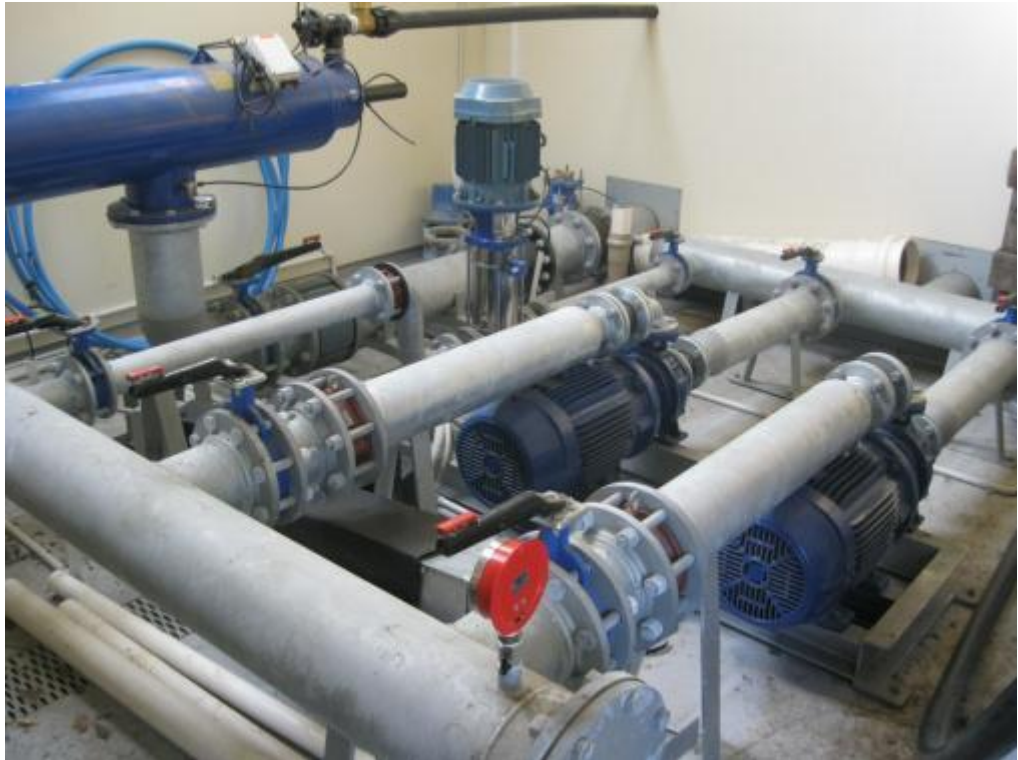
Photograph 5: Pumphouse equipment on reinforced concrete slab
