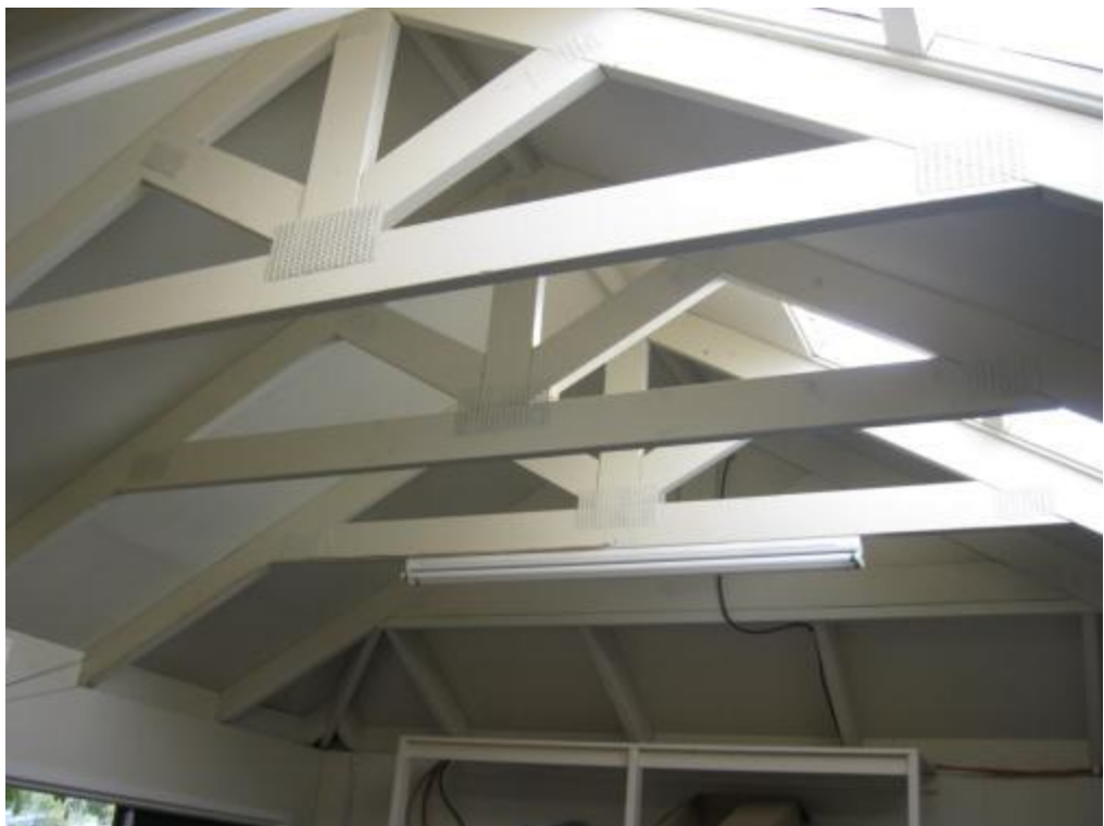
Photograph 4: Timber truss roof structure
