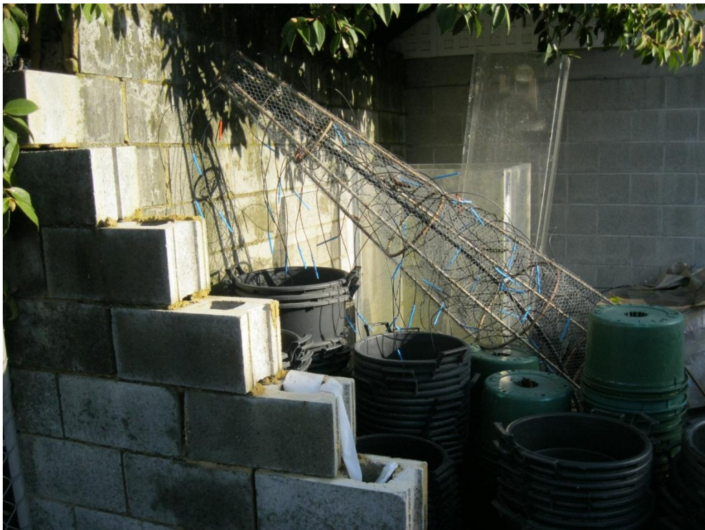
Photograph 8 Collapsed portion of the original wall.
