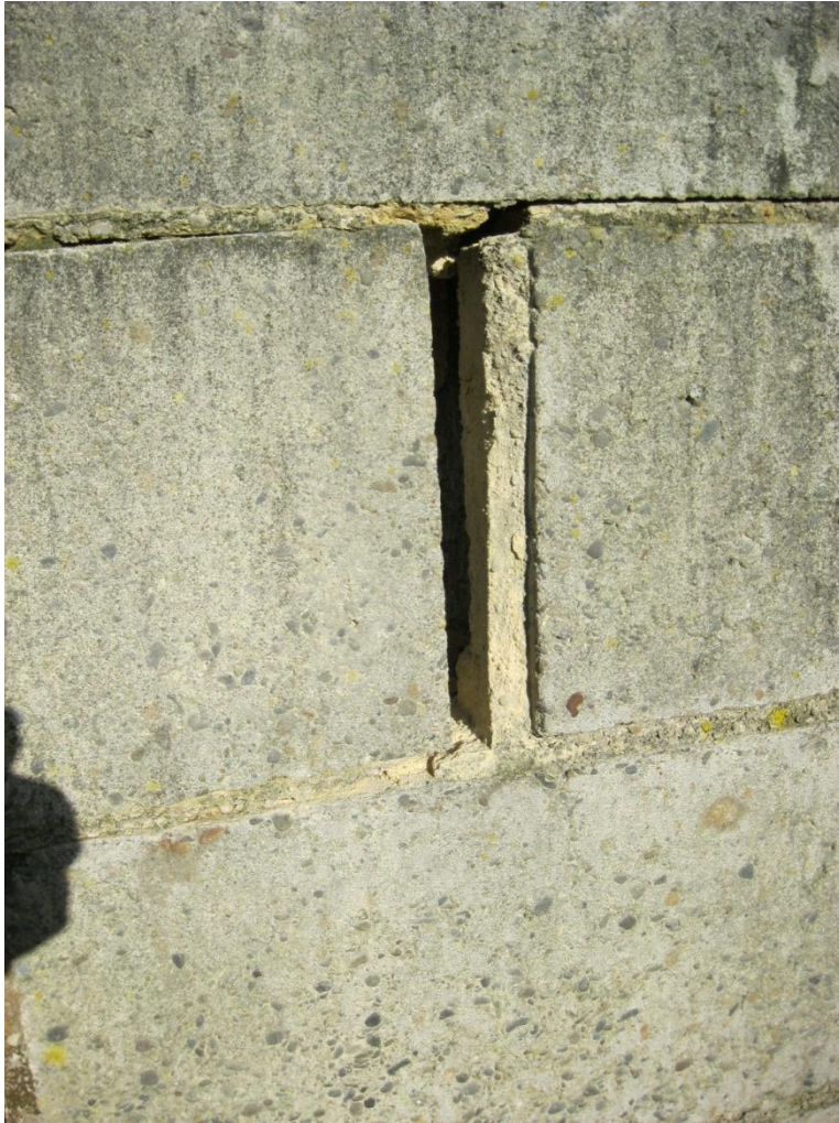
Photograph 9 Cracking to original wall away from the chemical store.
