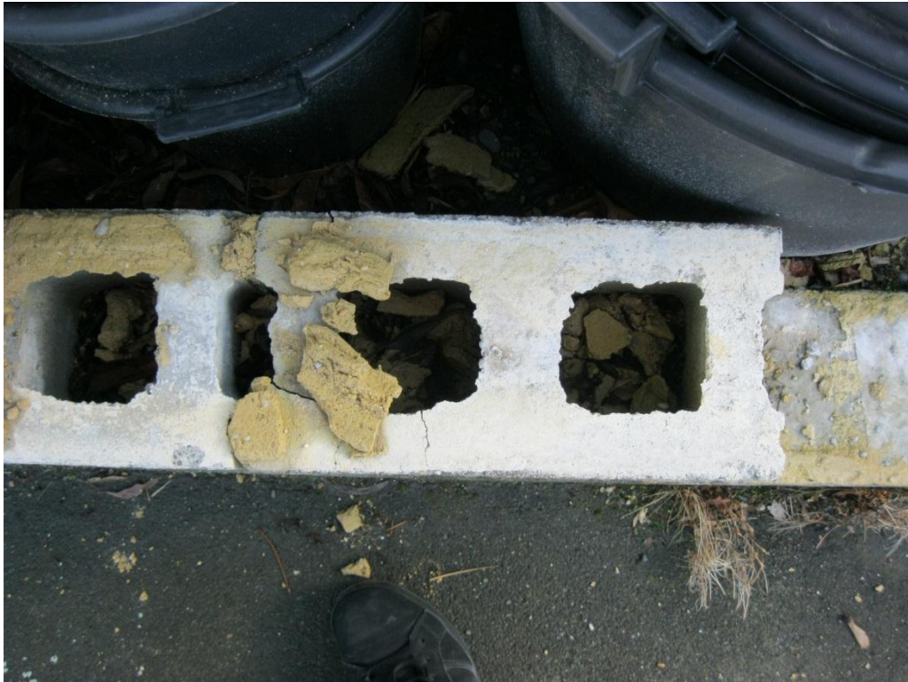
Photograph 7 Unfilled concrete masonry units of the collapsed portion of the original wall.
