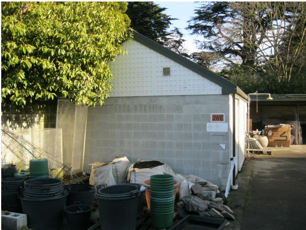
Photograph 4 The eastern face of the building.
