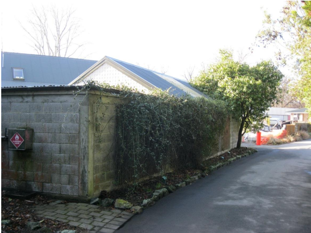
Photograph 3 The original southern wall of the building (Rear wall).
