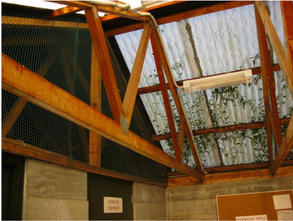
Photograph 5 Timber roof trusses and purlins visible. No roof cross-bracing present.
