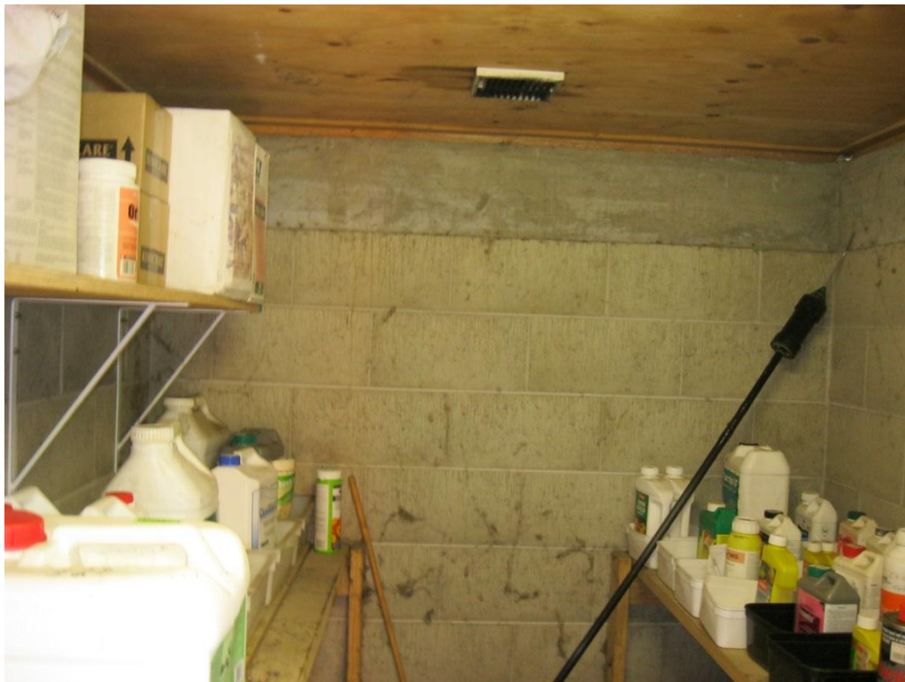
Photograph 6 Plywood ceiling lining to the underside of one of the rooms. A reinforced concrete ring beam is clearly visible.
