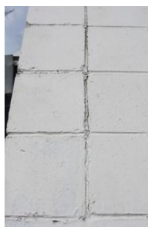
PHOTO 12: Detail of previous photo (probably earthquake damage)
