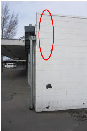
PHOTO 11: Side wall showing crack location
