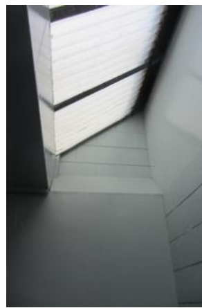
PHOTO 6: Interior view of hip roof
