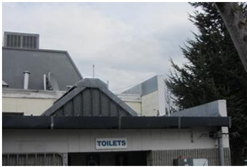
PHOTO 7: Exterior view of roof
