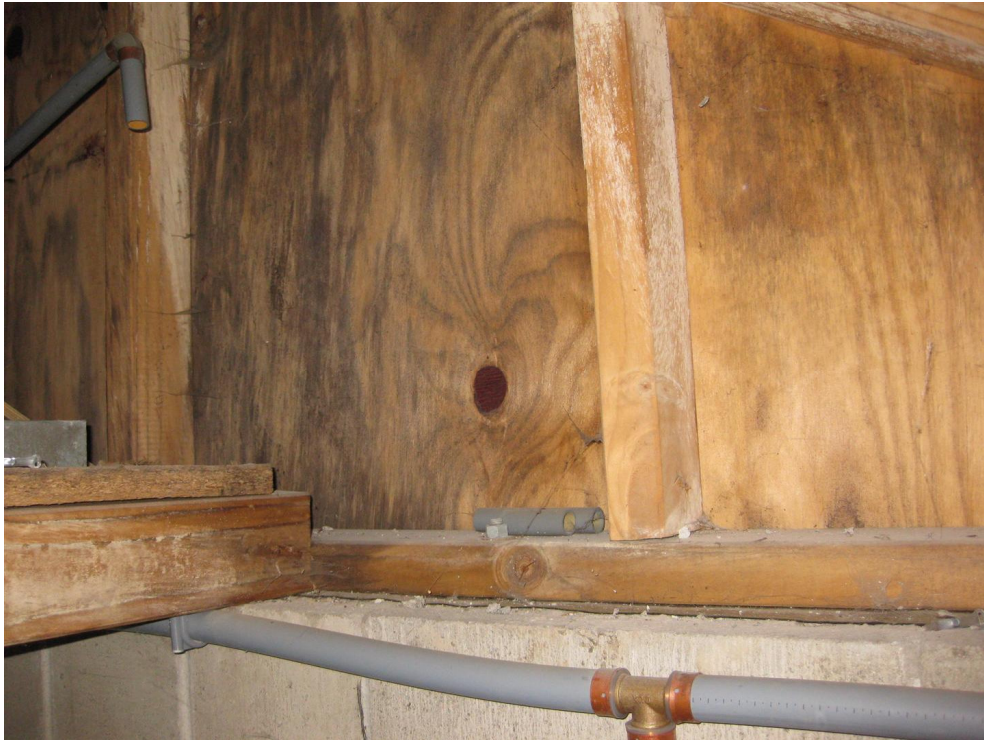
Photo 13: Internal timber to concrete block wall connection
