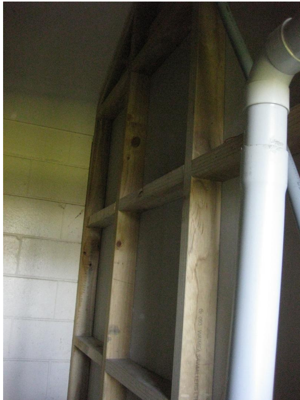
Photo 12: Internal timber partition wall
