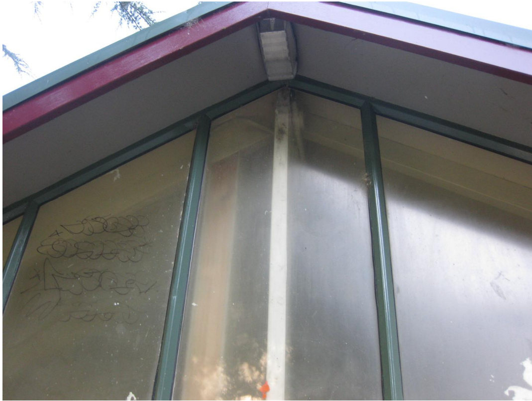
Photo 5: Exterior ridge detail
