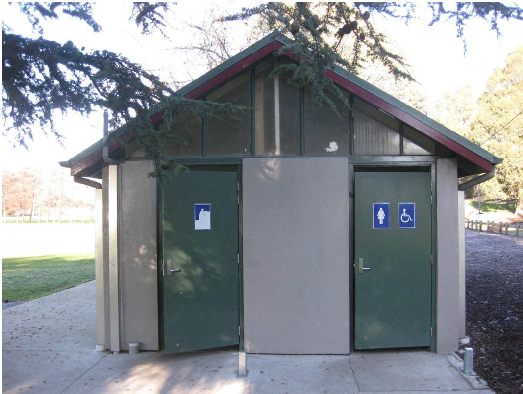
Photo 2: Side photo – female toilet entry
