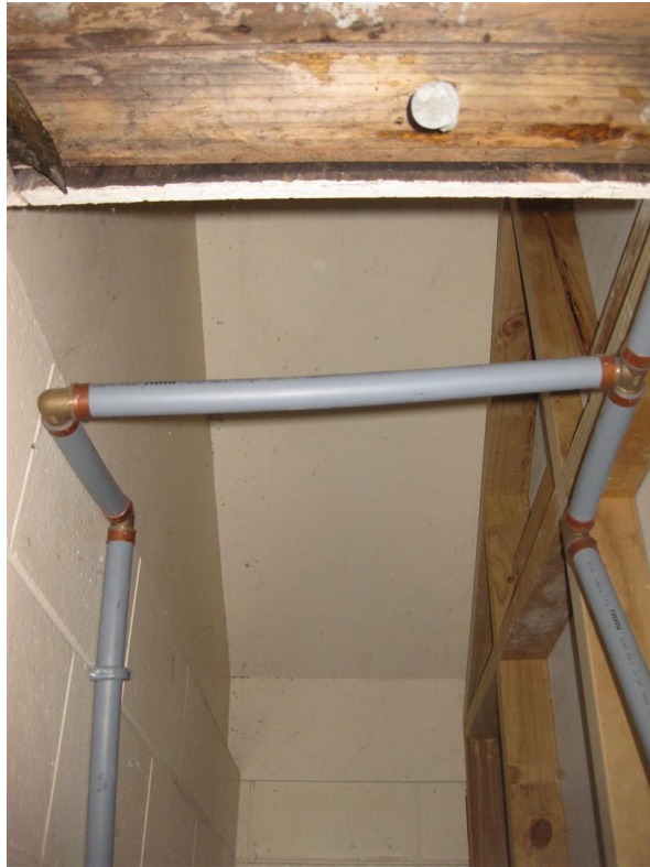
Photo 11: Internal concrete block and timber partition walls
