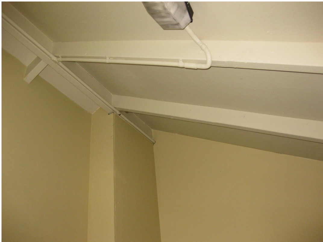
Photo 6: Interior ridge detail
