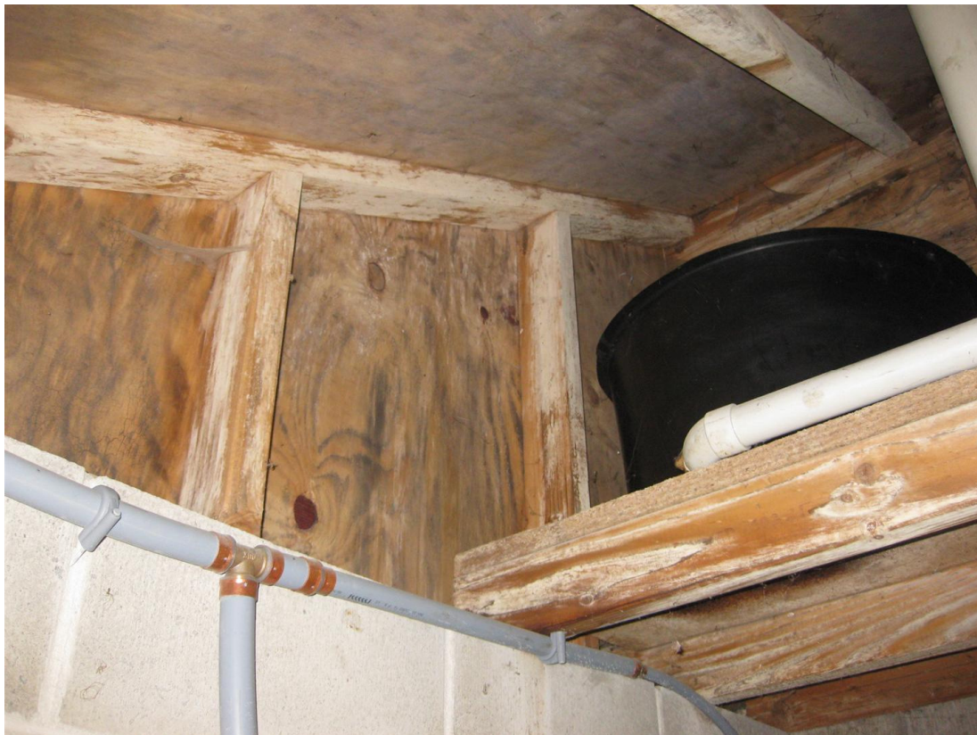
Photo 10: Timber partition wall on top of concrete block wall
