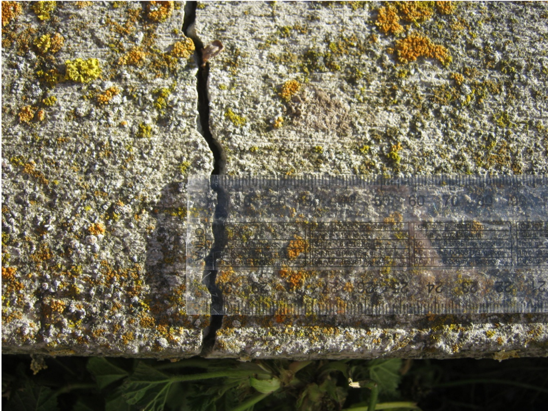
Photograph 11. 5mm crack across the southern concrete access ramp.
