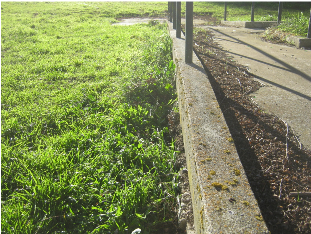
Photograph 12. Separation of 50mm between the ground and the front of the concrete access ramp.
