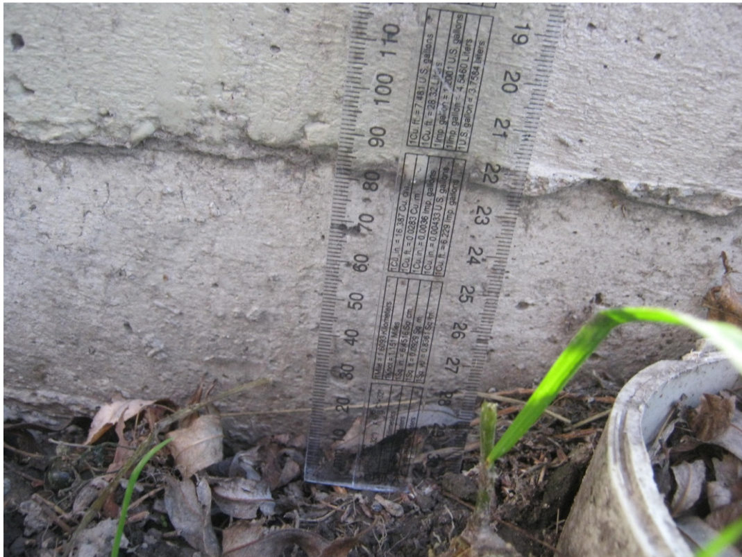
Photograph 9. The top of the perimeter strip footing 80mm above ground level at the northeast corner of the toilets.
