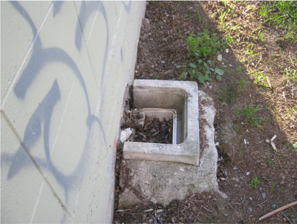
Photo 3: Separation of 30mm between the toilets and the concrete grey water collection box.
