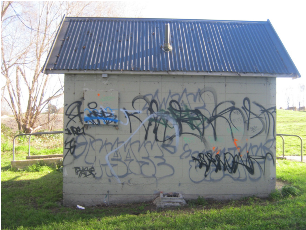
Photograph 3. Eastern Elevation, showing differential settlement from south to north.
