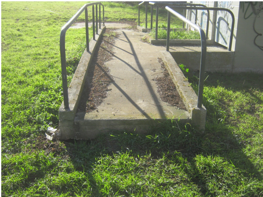
Photograph 10. Southern end of concrete access ramp.
