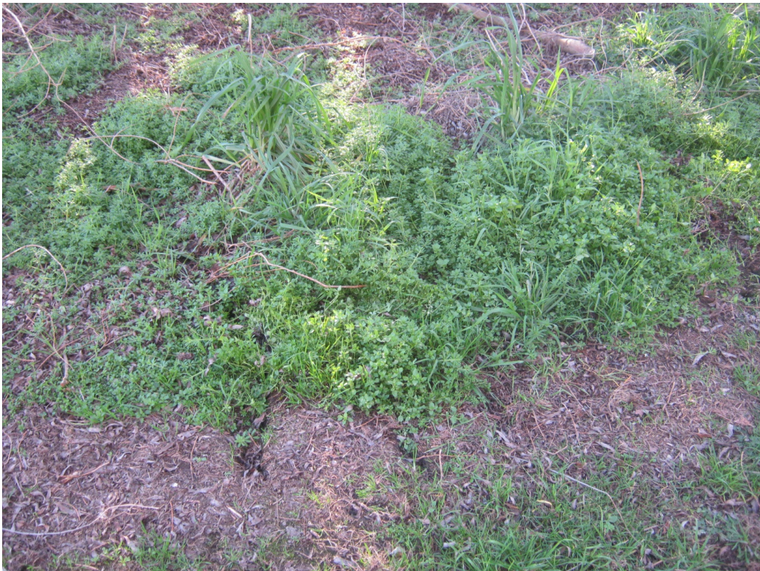
Photograph 18. Minor cracking about 15mm wide approximately 6m north of the toilets.
