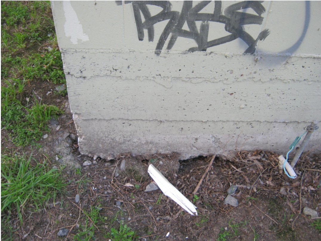
Photograph 15. Void underneath the south-western corner of the toilets.
