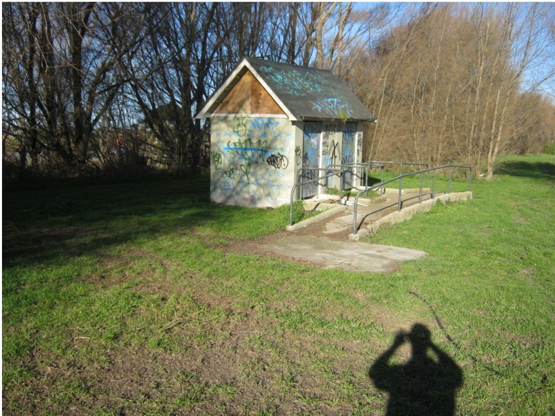
Photograph 7. Ejected sand from liquefaction adjacent to the toilets.
