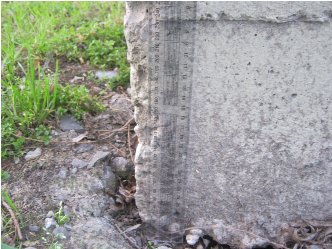
Photograph 8. The top of the perimeter strip footing 230mm above ground level at the southeast corner of the toilets.
