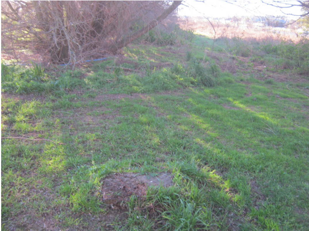
Photograph 17. Manhole adjacent to the toilets that appears to have risen by approximately 100mm.
