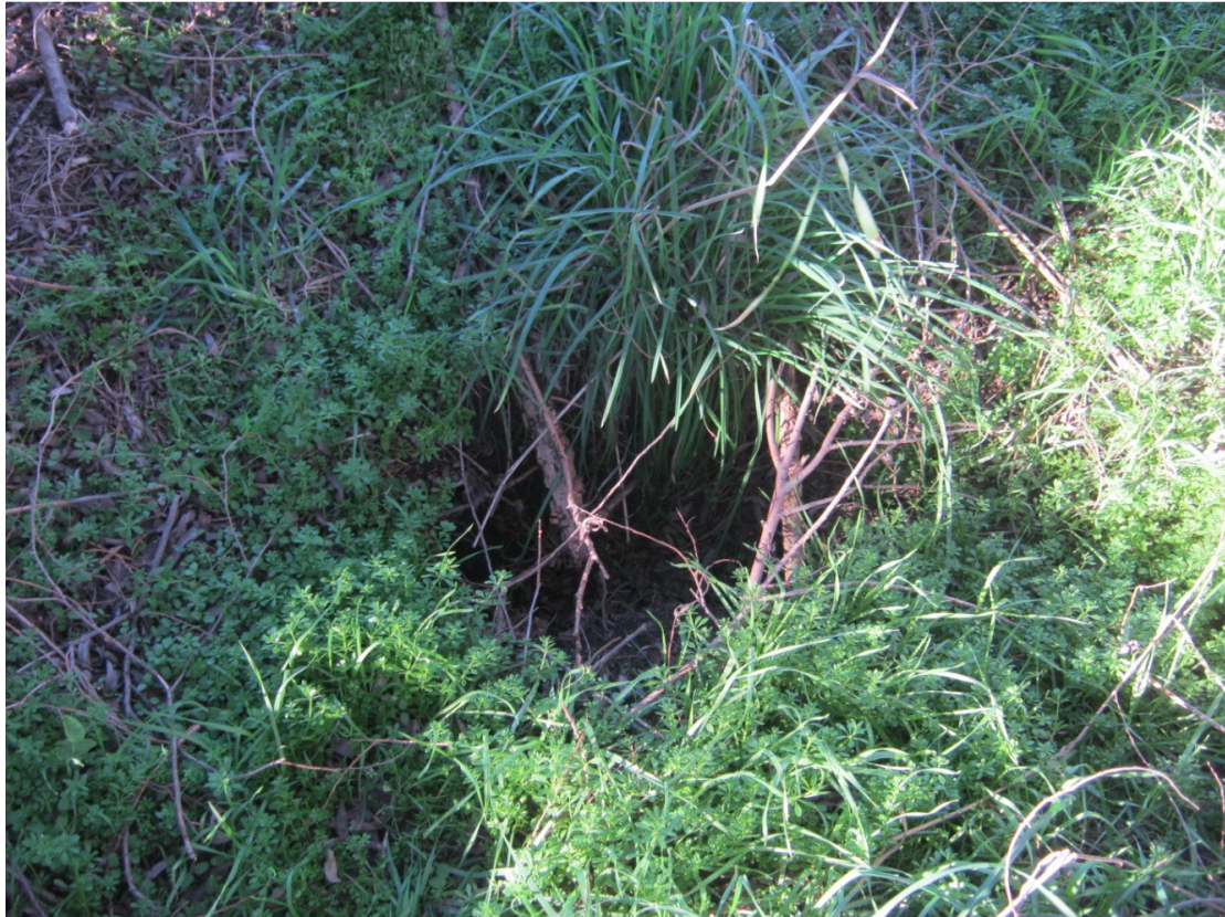
Photograph 19. Collapsed void approximately 500mm wide in the tree line to the east of the toilets.
