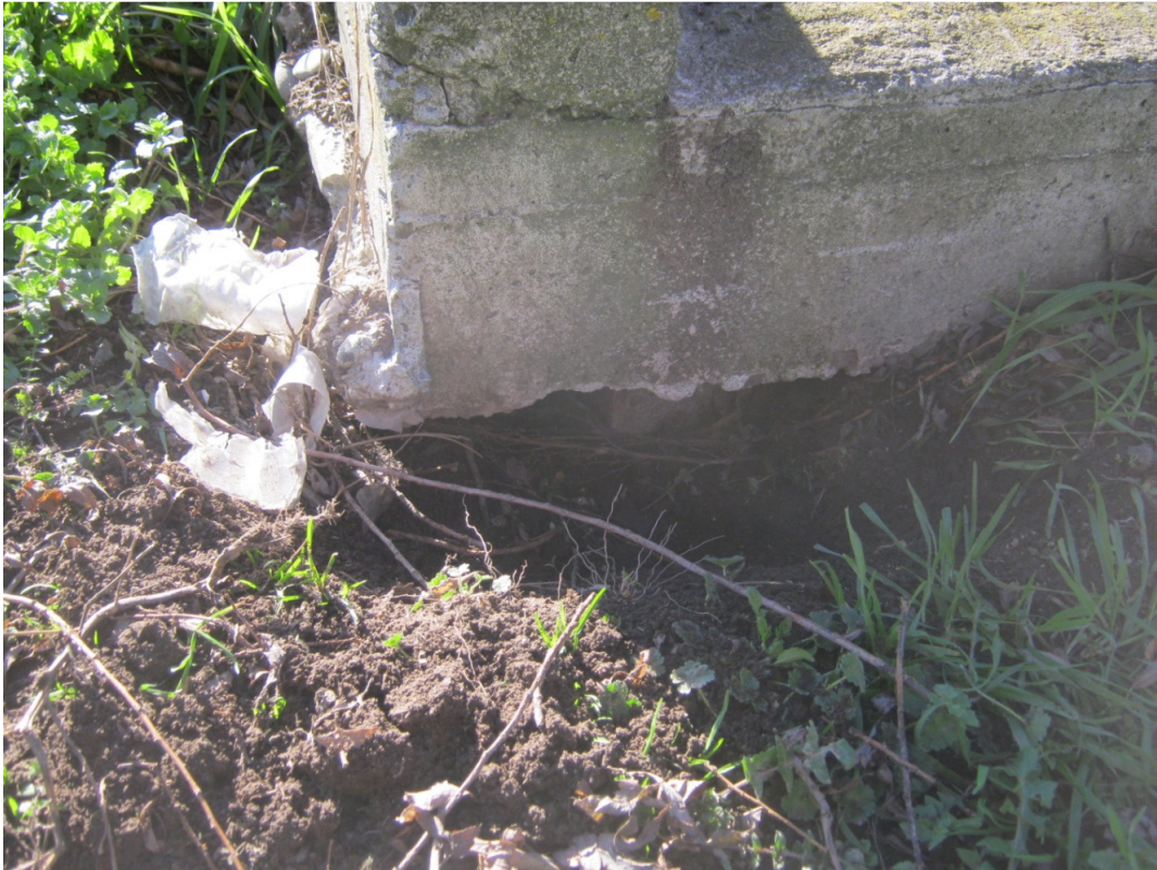
Photograph 13. Void underneath the south-western corner of the concrete access ramp.
