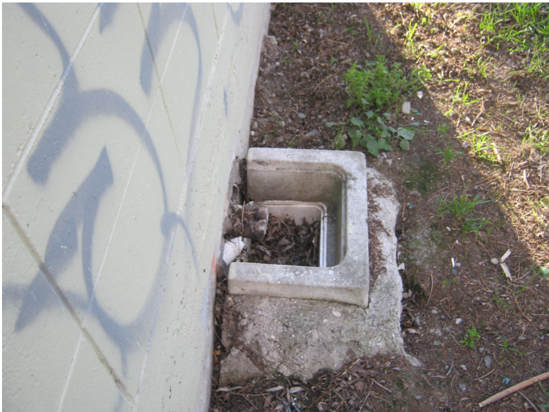
Photograph 16. Separation of 30mm between the toilets and the concrete grey water collection box.
