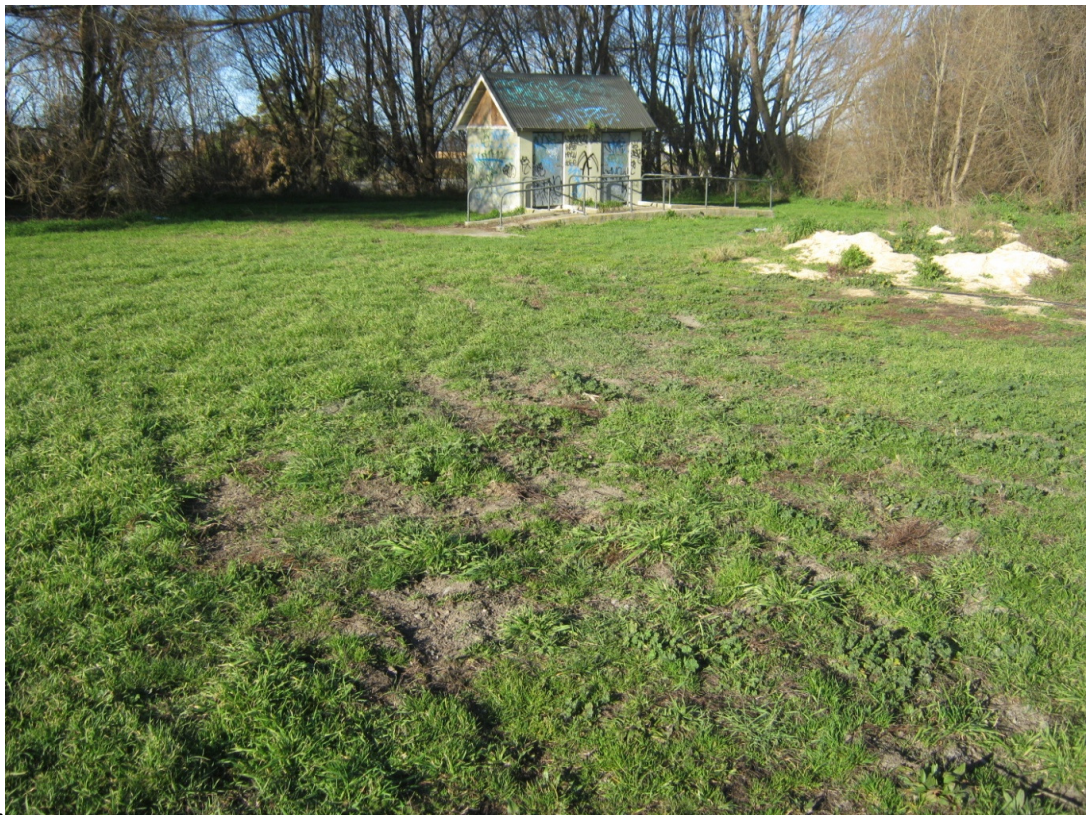
Photograph 6. Ejected sand from liquefaction on the grassed area to the east of the toilets.
