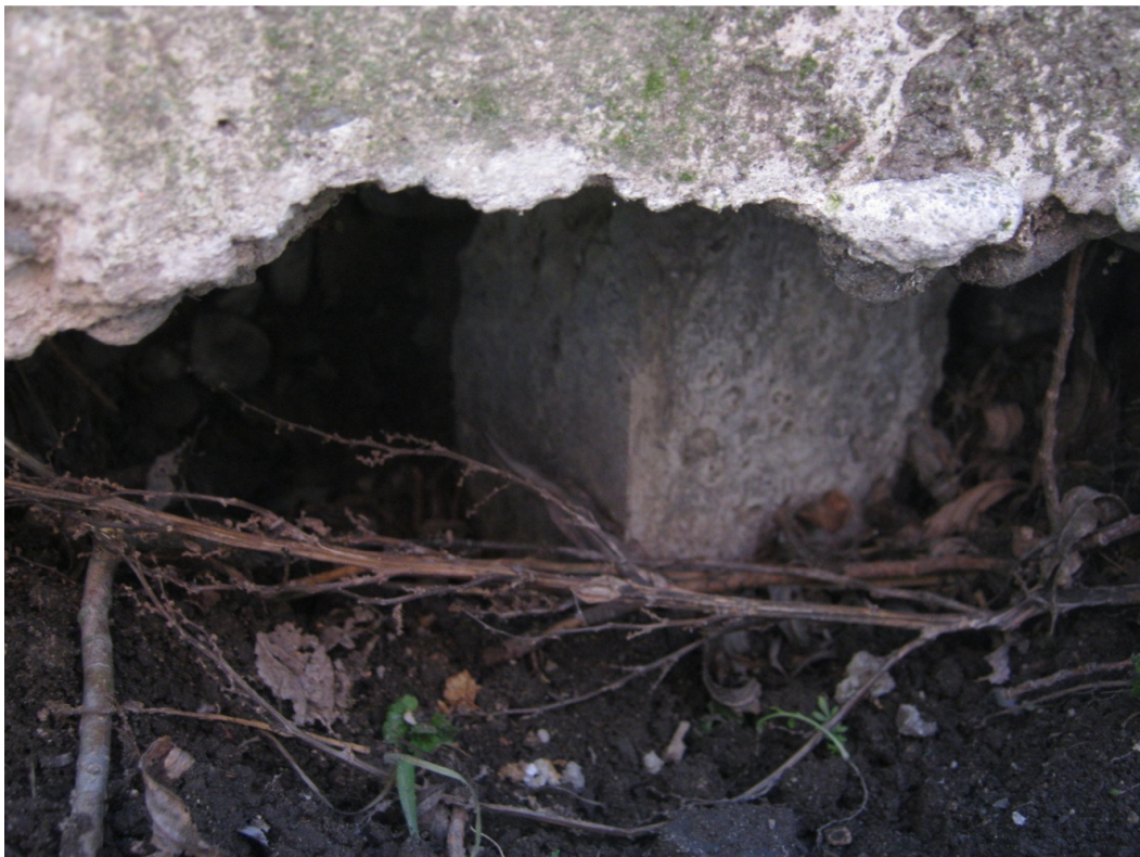
Photograph 14. A pile within the void under the south-western corner of the concrete access ramp.
