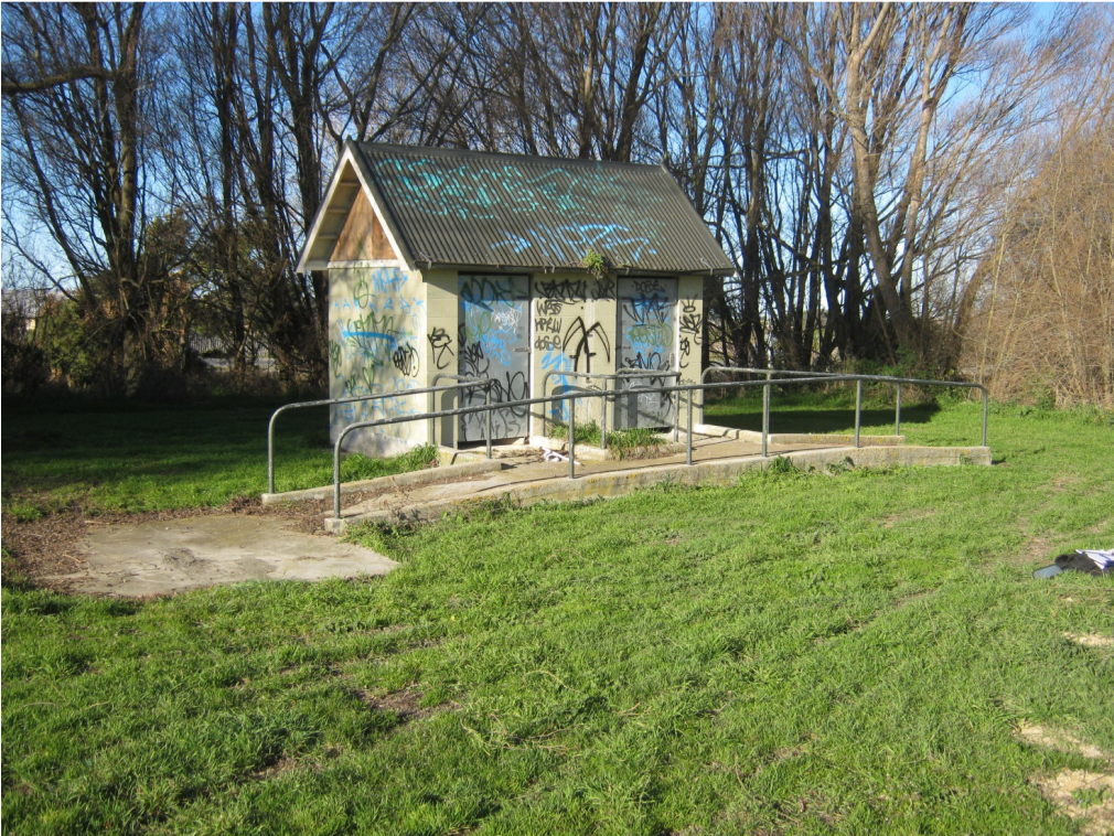
Photo 1: The north and west wall of the building.
