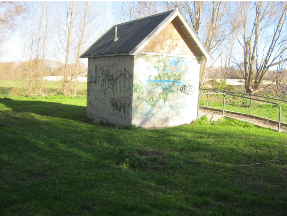
Photo 2: The north and east wall of the building.
