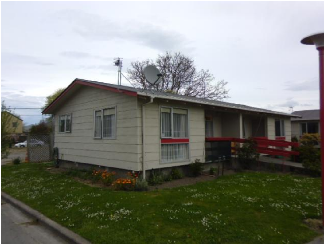
Photograph 1 View of Block A
