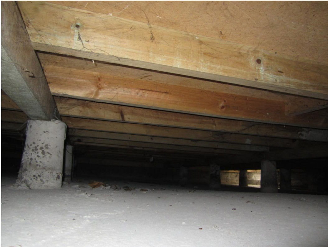
Photograph 11 View of foundations of Block F
