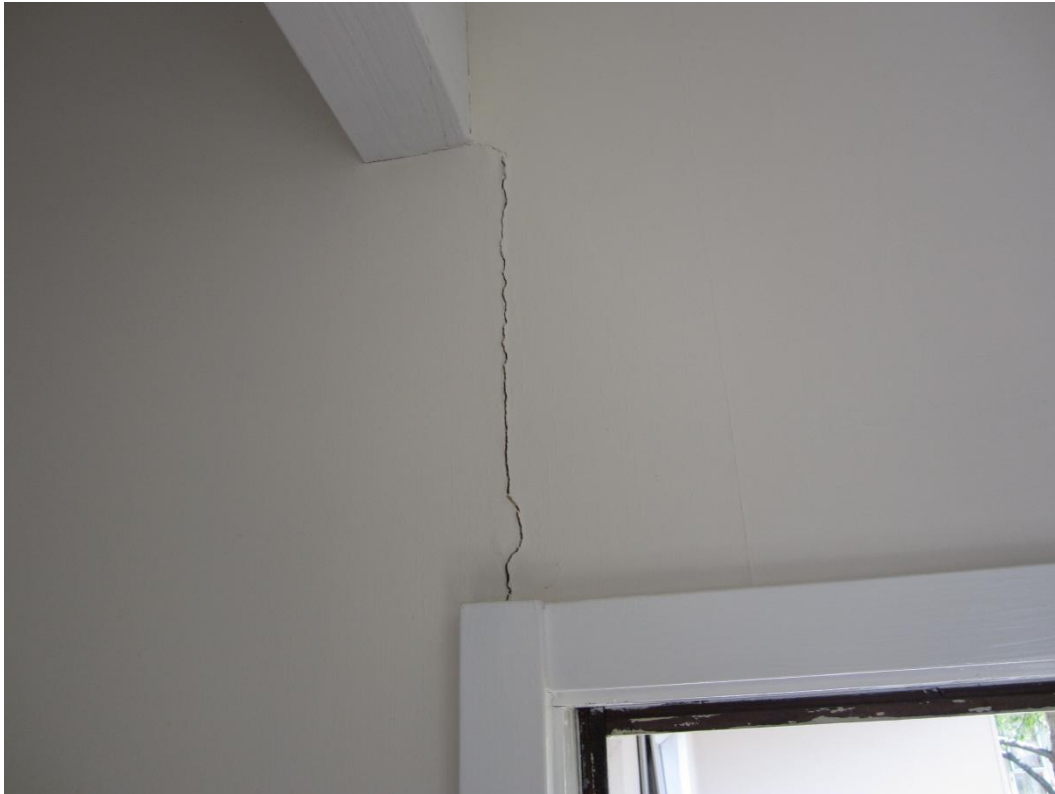
Photograph 5 Cracking between timber lintel and corner of window in Block B
