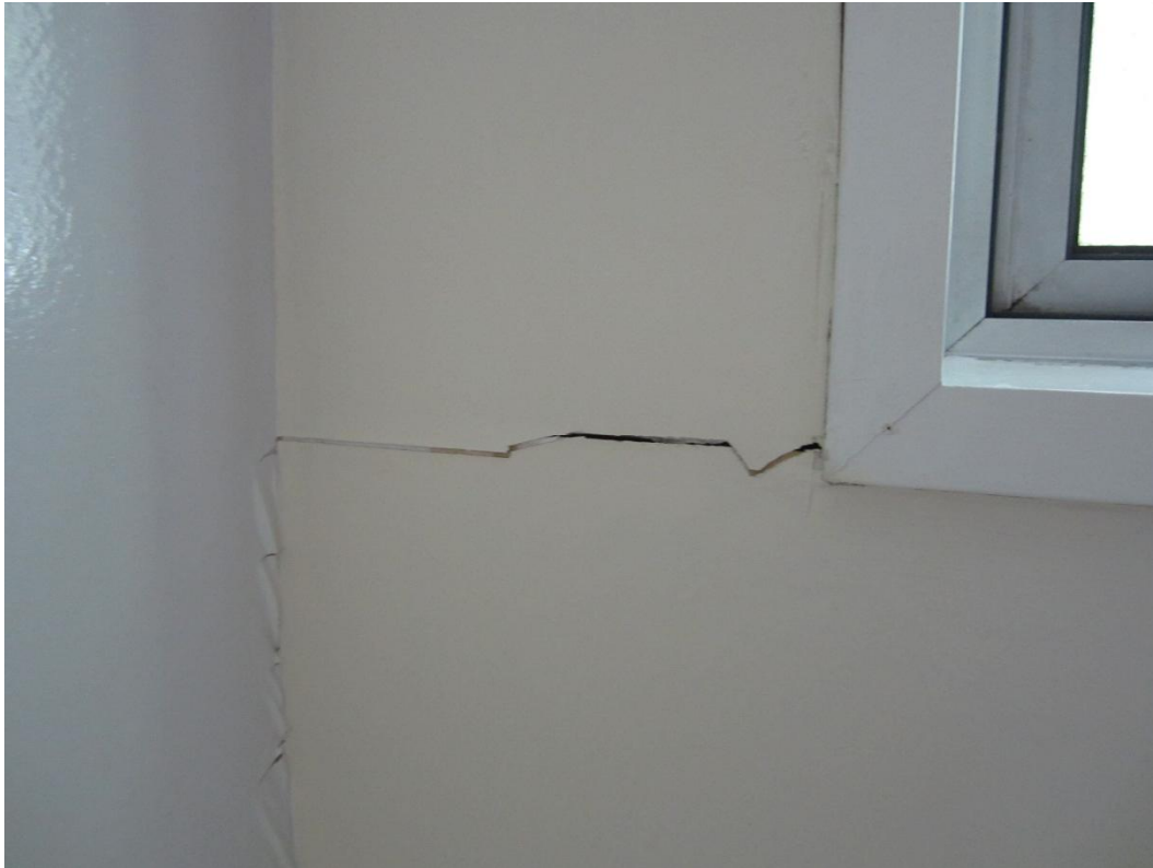
Photograph 3 Cracking at corner of window in Block A
