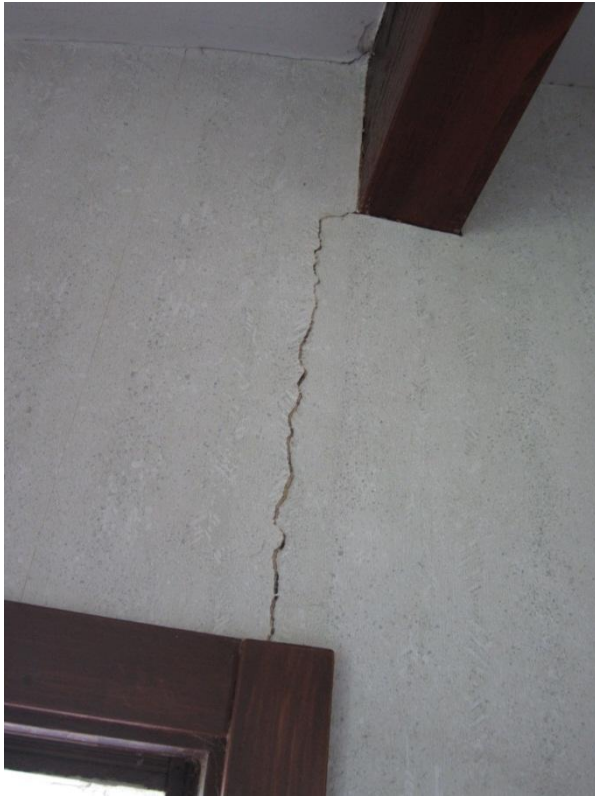
Photograph 7 Cracking between timber lintel and corner of window in Block C
