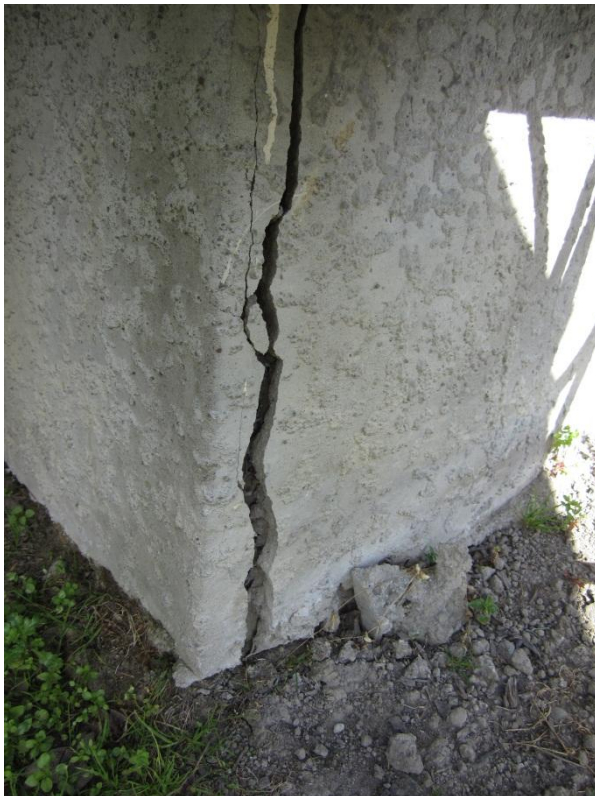
Photograph 2 Cracking to corner of concrete foundation wall in Block A
