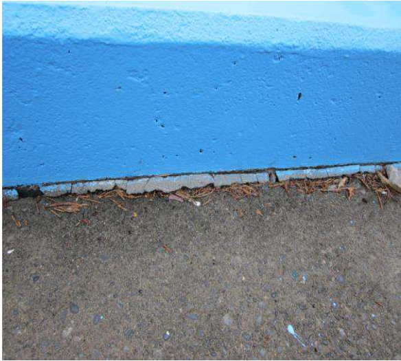
Concrete slab pulling away from edge of pool
