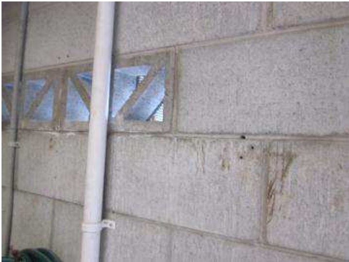
Diagonal cracking on internal wall in women's changing room (West End)
