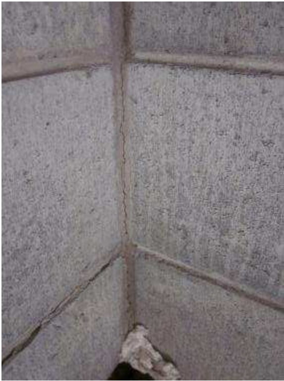
Cracking on interior corners of building in men's changing room (East end)
