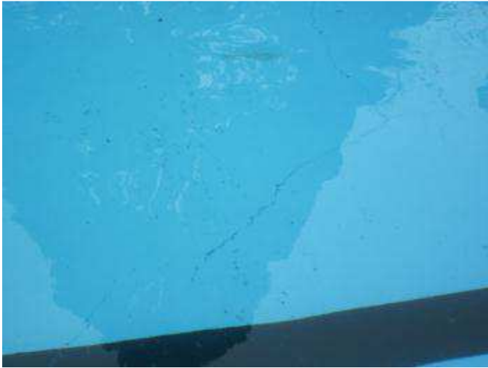
Cracking on base of pool
