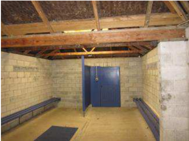
No noticeable damage to light timber roof frames
