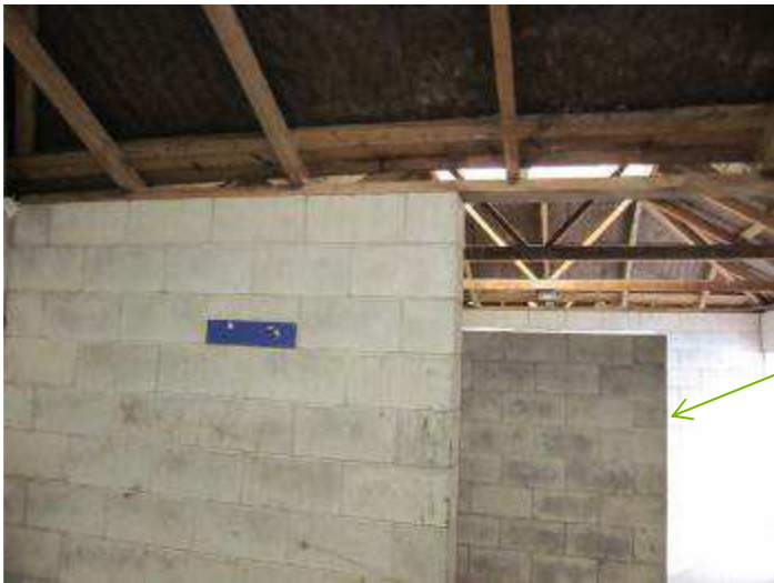
Potential fall hazard of hollow internal walls.
