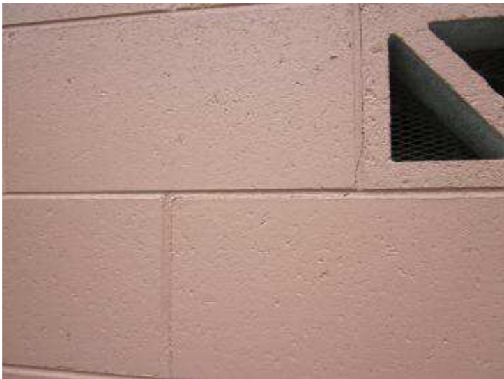
Cracking on external southern wall.
