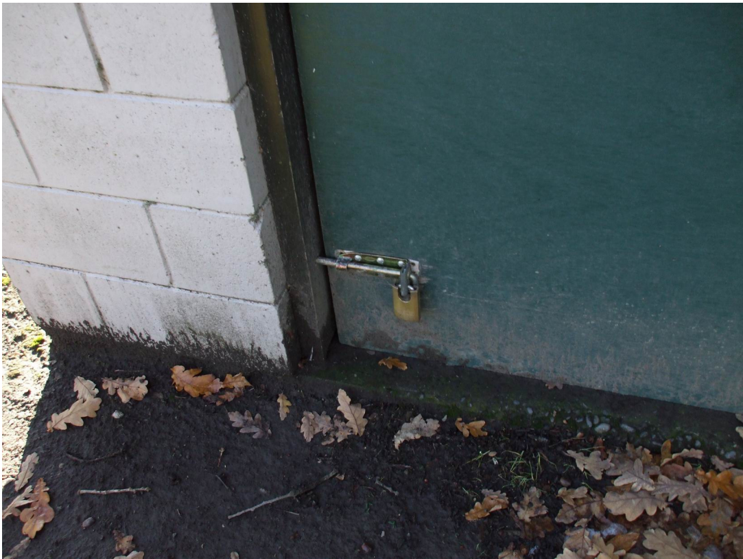
Photo 6: Bottom at garage door
