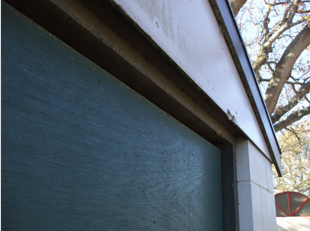
Photo 5: Top of garage door
