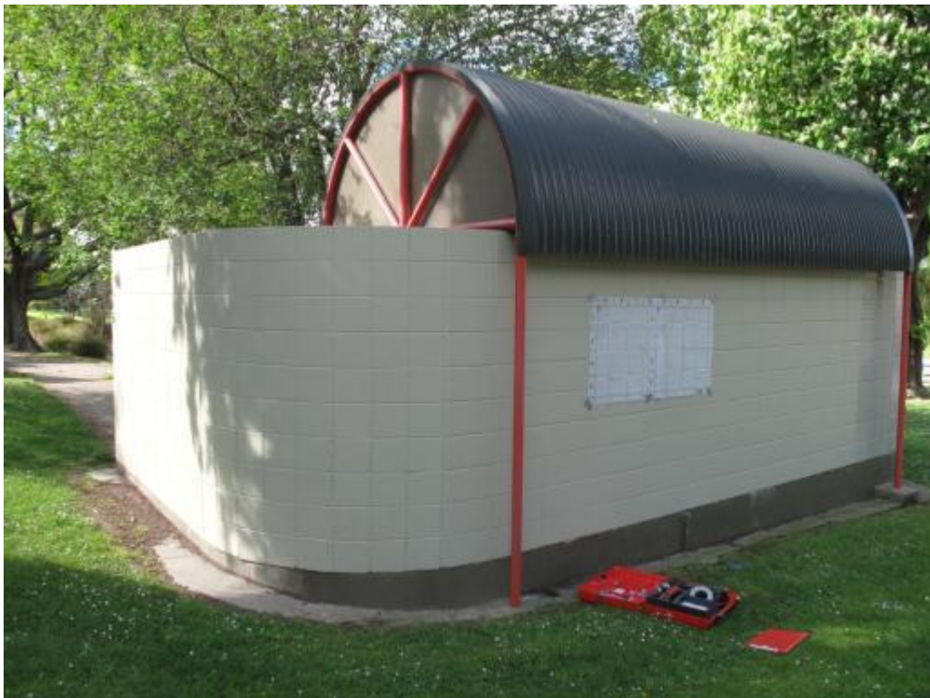
Photograph 10 Area of rear wall where reinforcement checks have been done.
