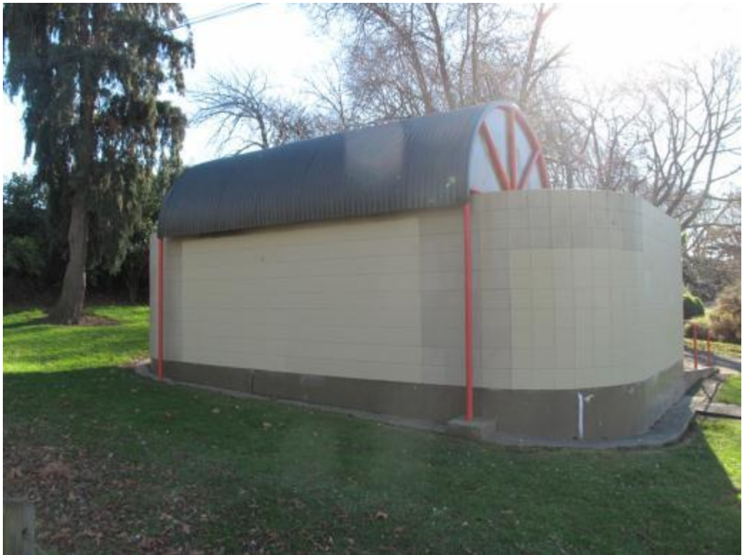
Photograph 2 View of the toilet block from the south.
