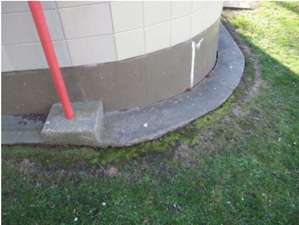
Photograph 5 Minor damage to the base where the strip footings have settled.
