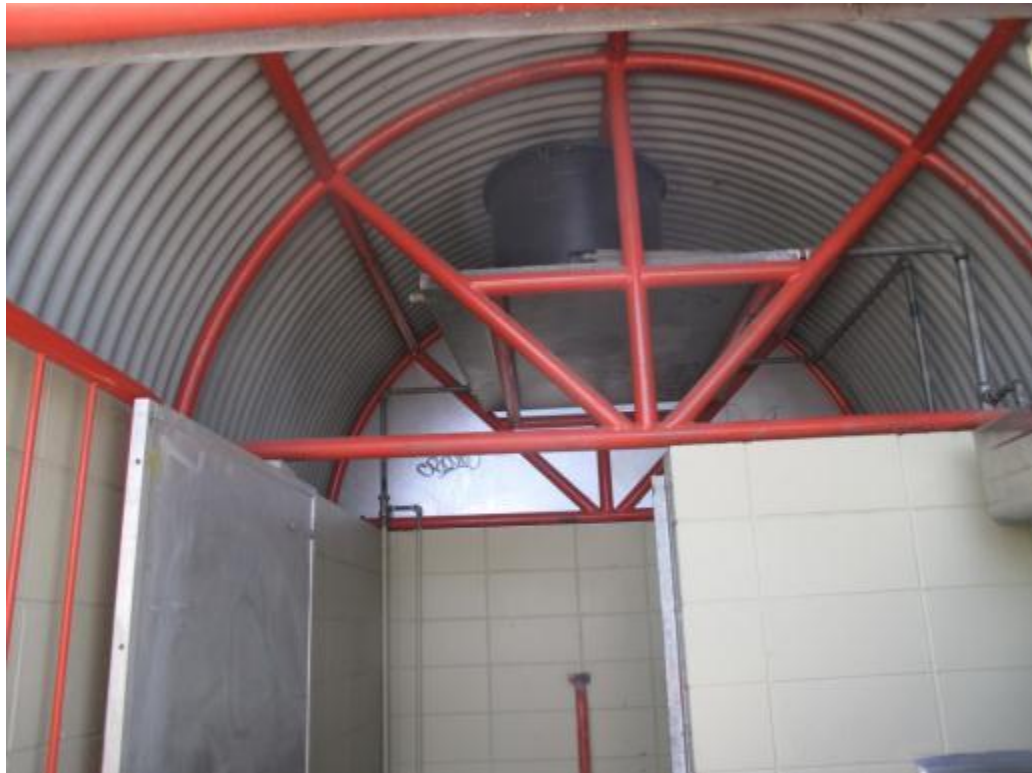
Photograph 7 Steel trusses and welded structure.
