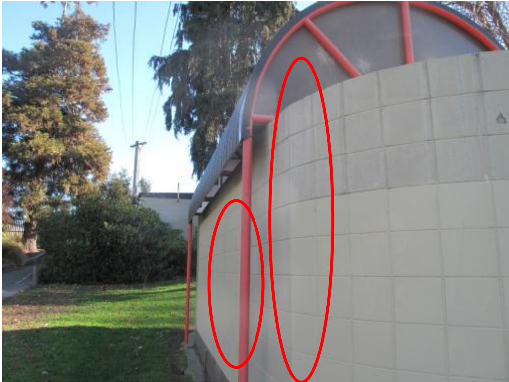
Photograph 9 Roof structure is largely supported by four steel posts.
