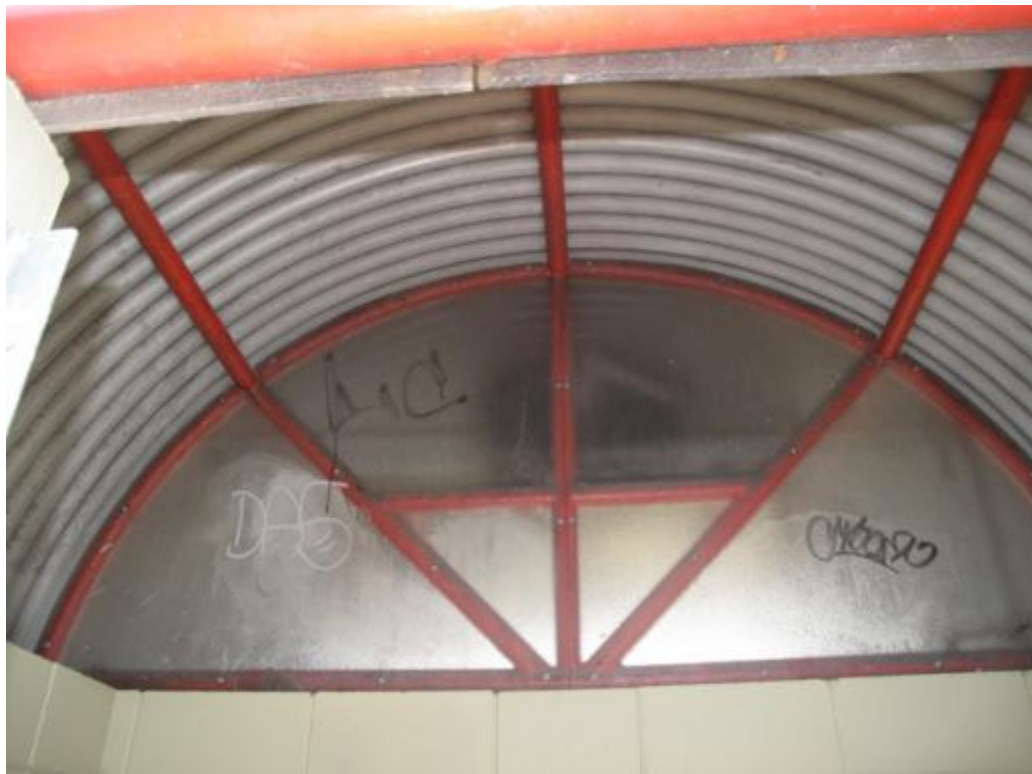
Photograph 8 Edge of roof structure with steel truss.
