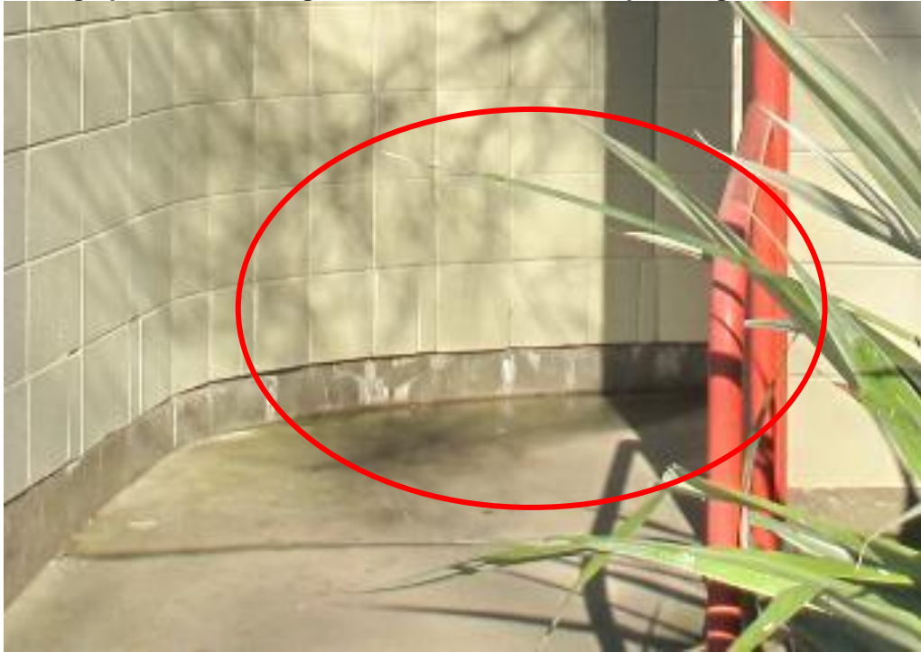
Photograph 5 Minor damage to the base where the strip footings have settled.
