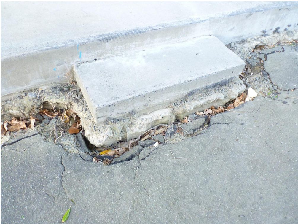
Displacement at front steps
