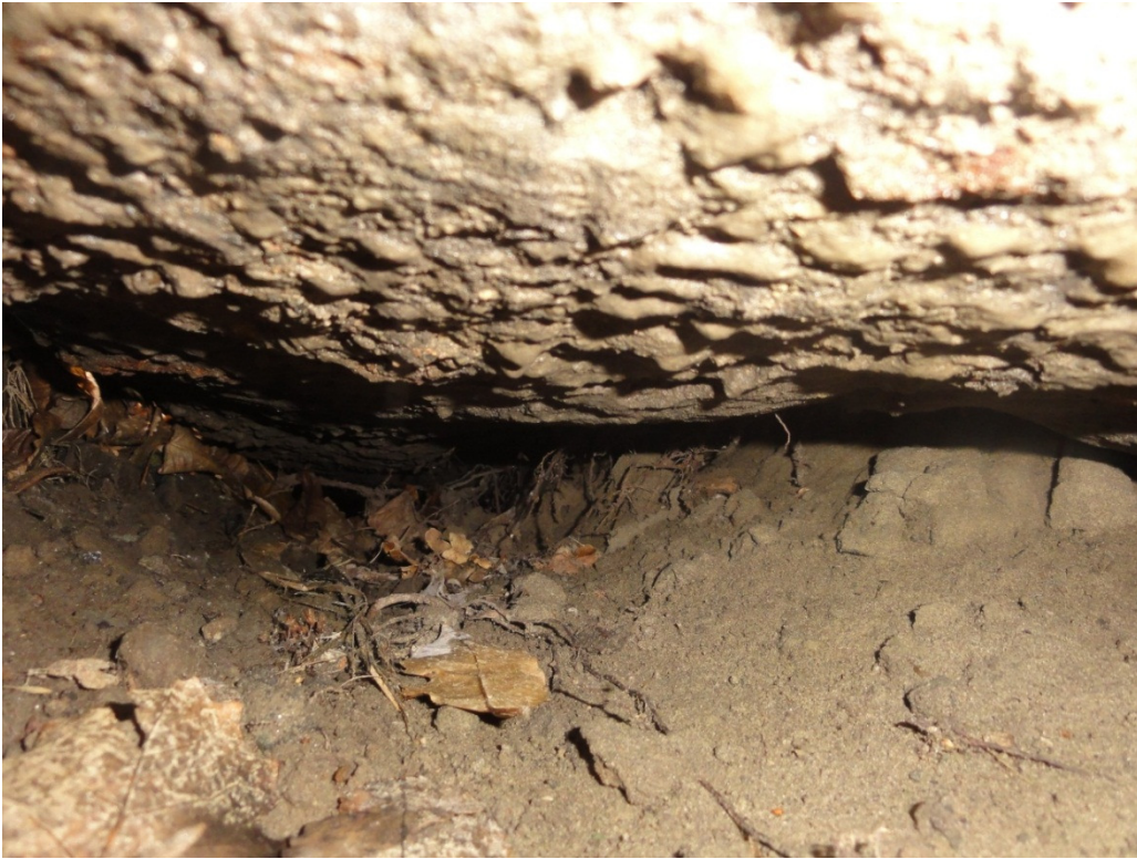
Figure 5: Void underneath the south eastern corner of the concrete floor slab.
