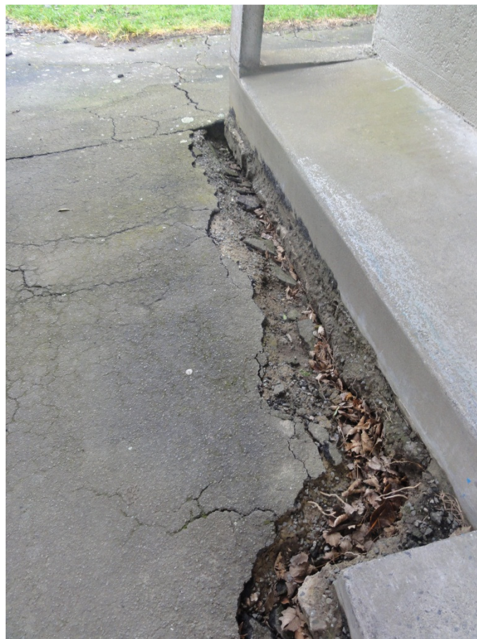
Figure 4: Ground deformation on the south eastern corner of the building.
