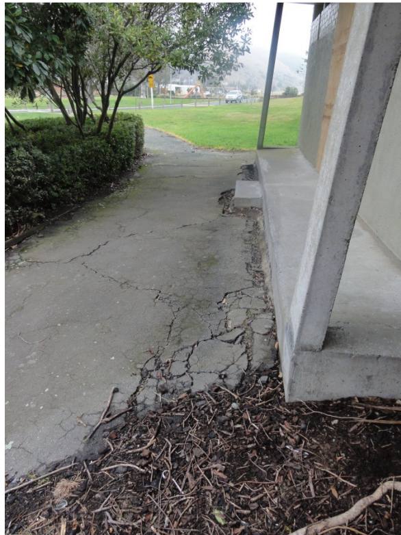
Figure 3: Asphalt damage along the eastern side of the building.
