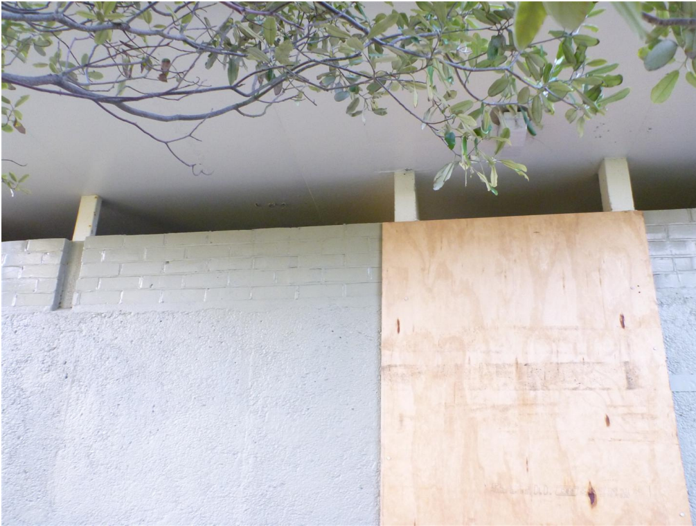
West wall. Note: Concrete wall not full height to roof diaphragm
