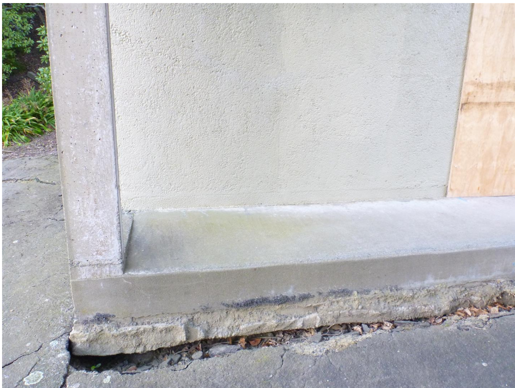
Pavement damage indicating movement of toilet facility
