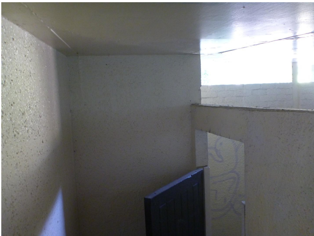
Interior 0.9m full-height north-south wall – the only north-south wall that is full-height
