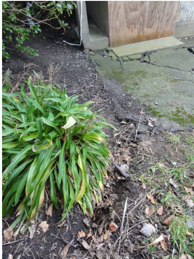
Figure 6: Tension crack extending from the south western corner of the building.
