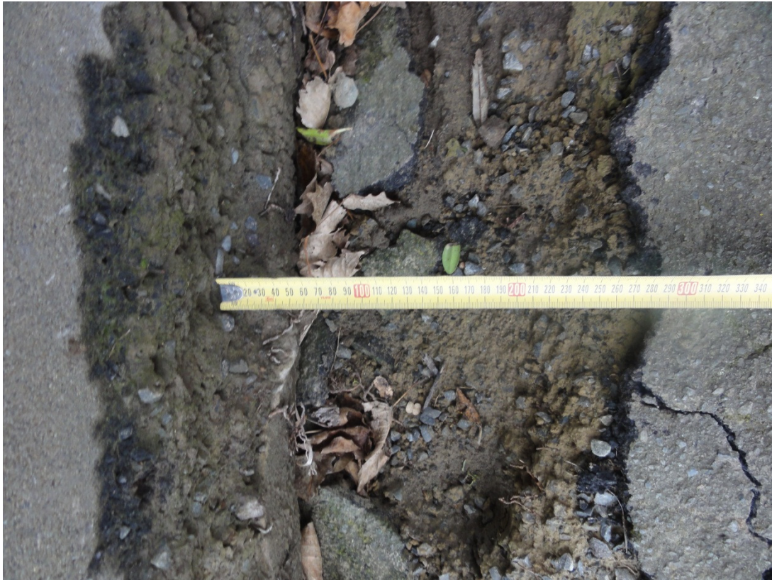
Figure 7: the asphalt along the eastern side has been offset by approximately 300mm.
