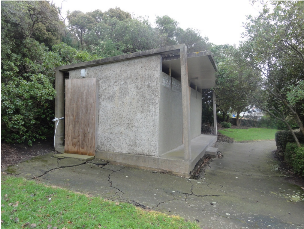
Figure 1: Southern elevation of the Barnett Park Toilet building.
