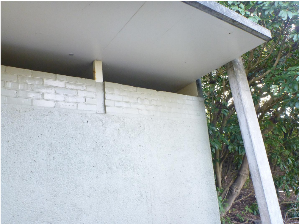
North and west faces of Barnett Park Toilets
