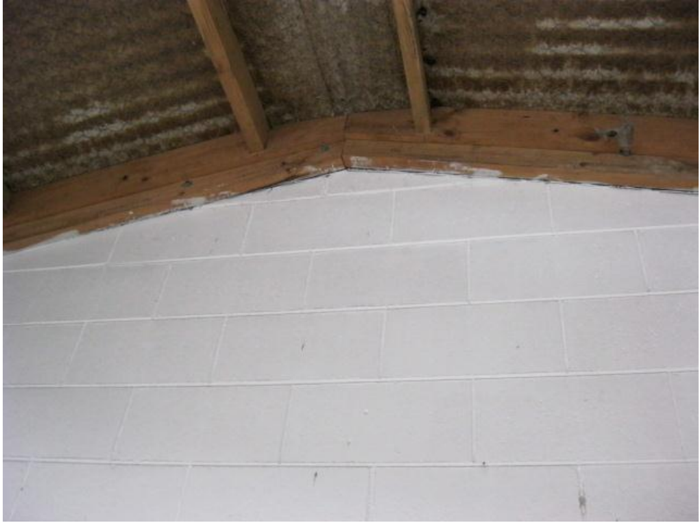
Photograph 9 Masonry walls extending the full height of the building to roof apex level.
