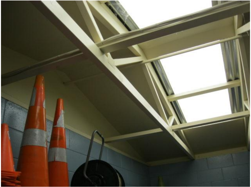
Photograph 5 Timber roof trusses of referee changing room/equipment storage building.
