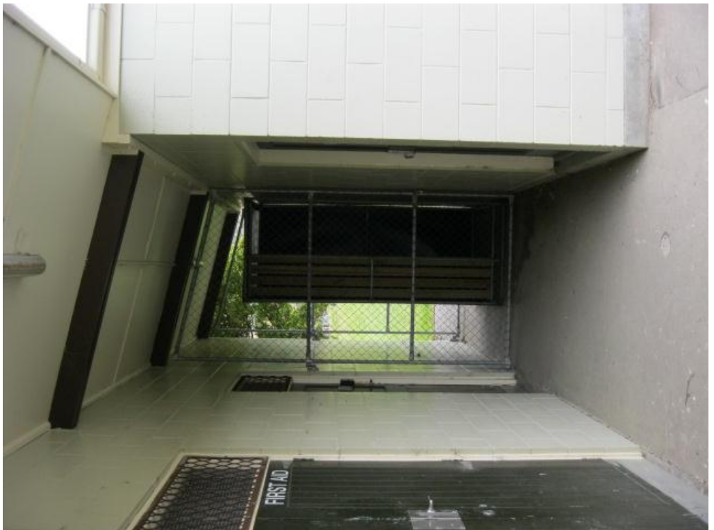
Photograph 6 Gap between sections of the building.
