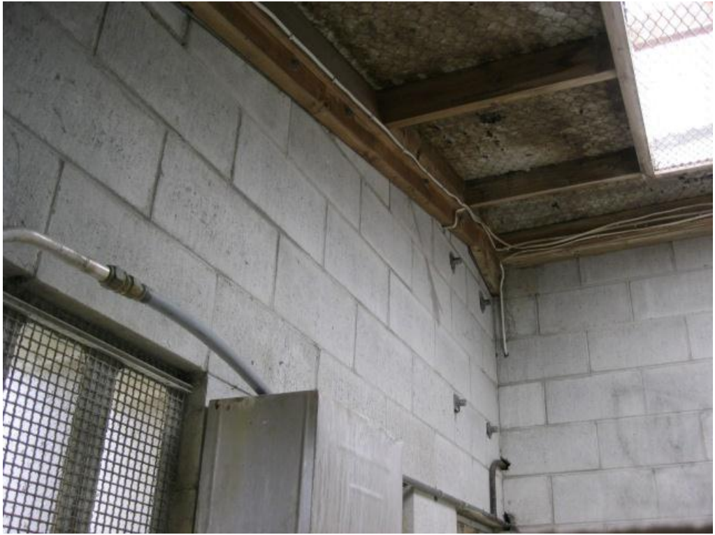
Photograph 7 Roof of toilet block/changing rooms.
