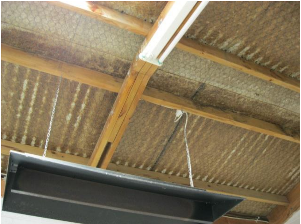
Photograph 8 Roof cladding, timber purlins and timber rafters in the roof of the toilet block/changing rooms.
