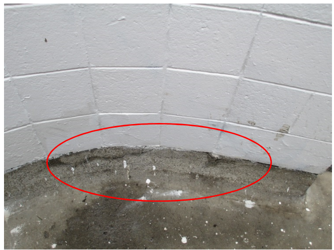
Cracks in the connection of the walls with the concrete foundation.
