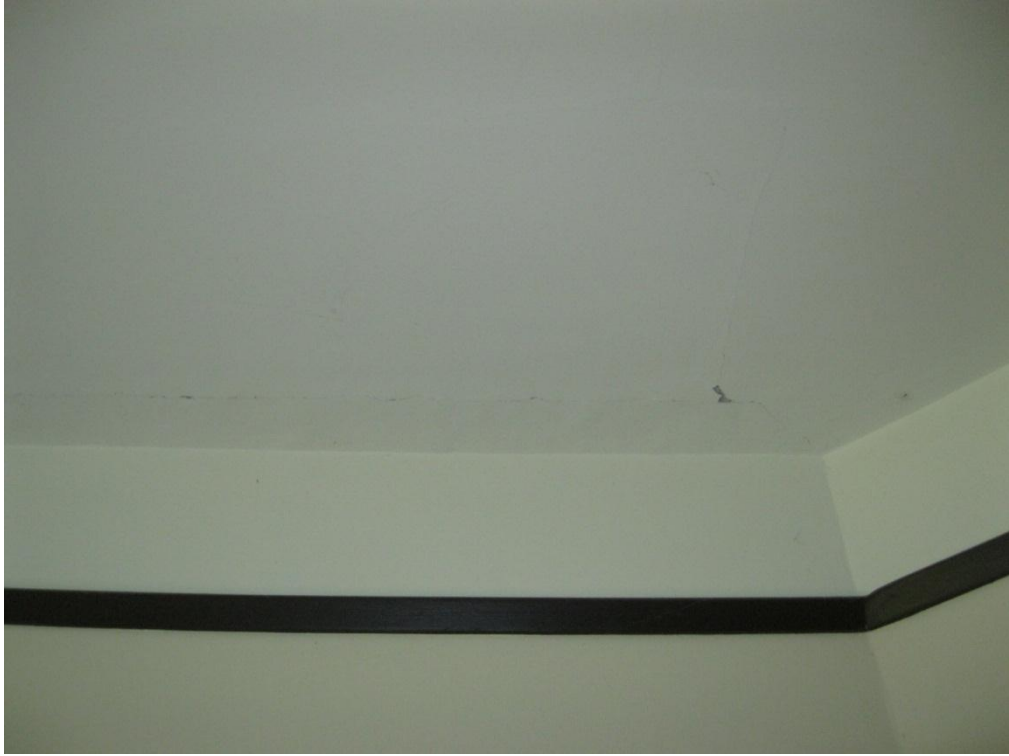
Photograph 7 Cracking to plasterboard ceiling lining.
