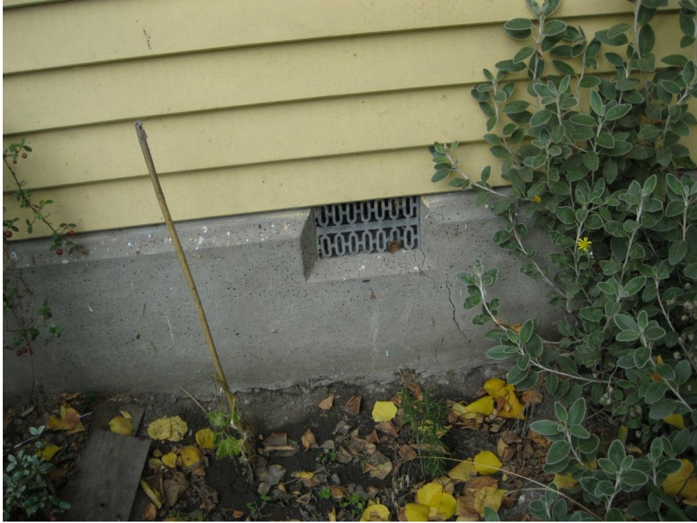
Photograph 9 Cracking to concrete perimeter strip foundation.
