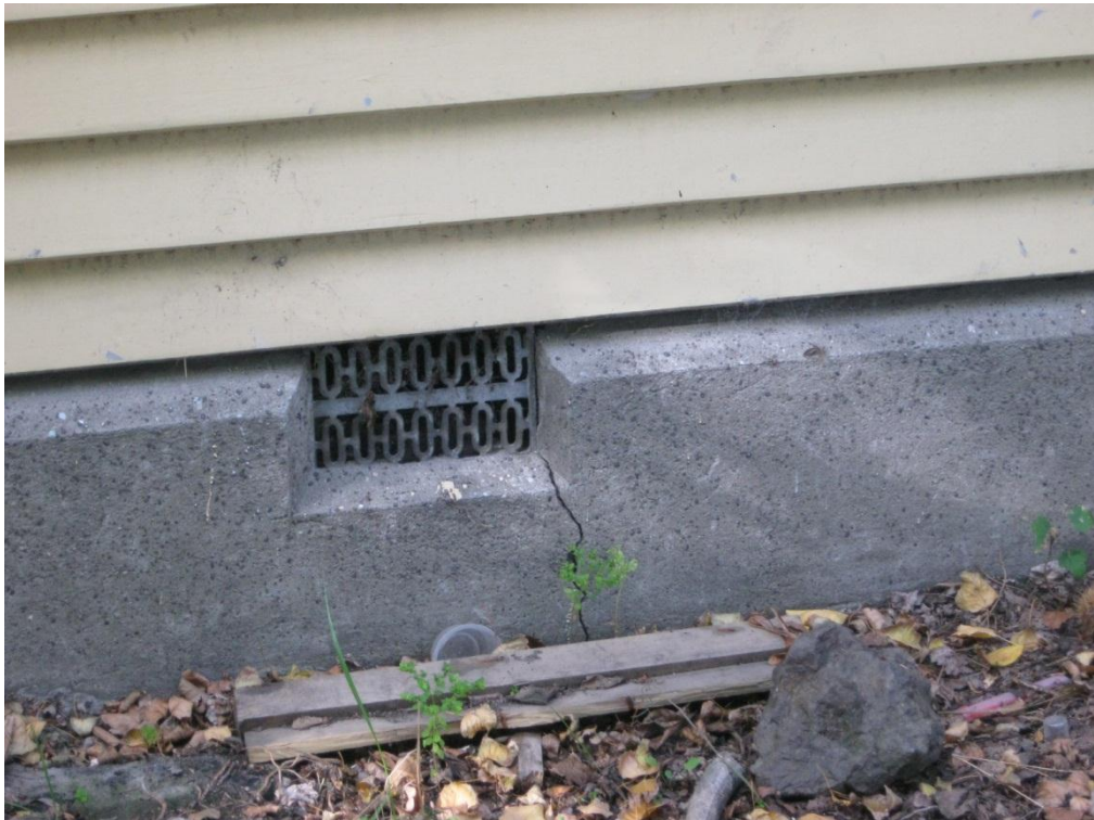
Photograph 9 Cracking to concrete perimeter strip foundation.
