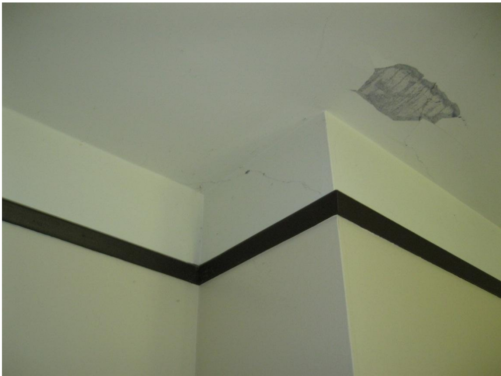
Photograph 7 Cracking to plasterboard ceiling lining.
