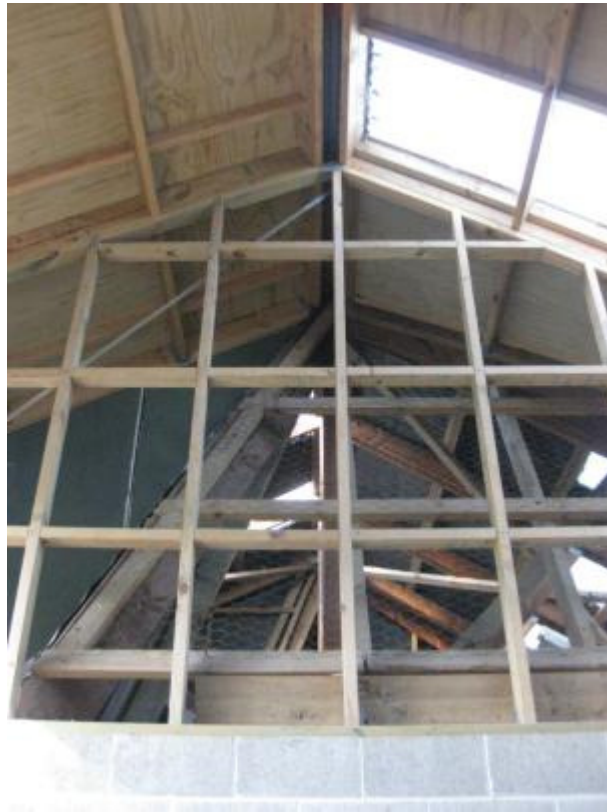
Photo 3: Ceiling diaphragm in extension
