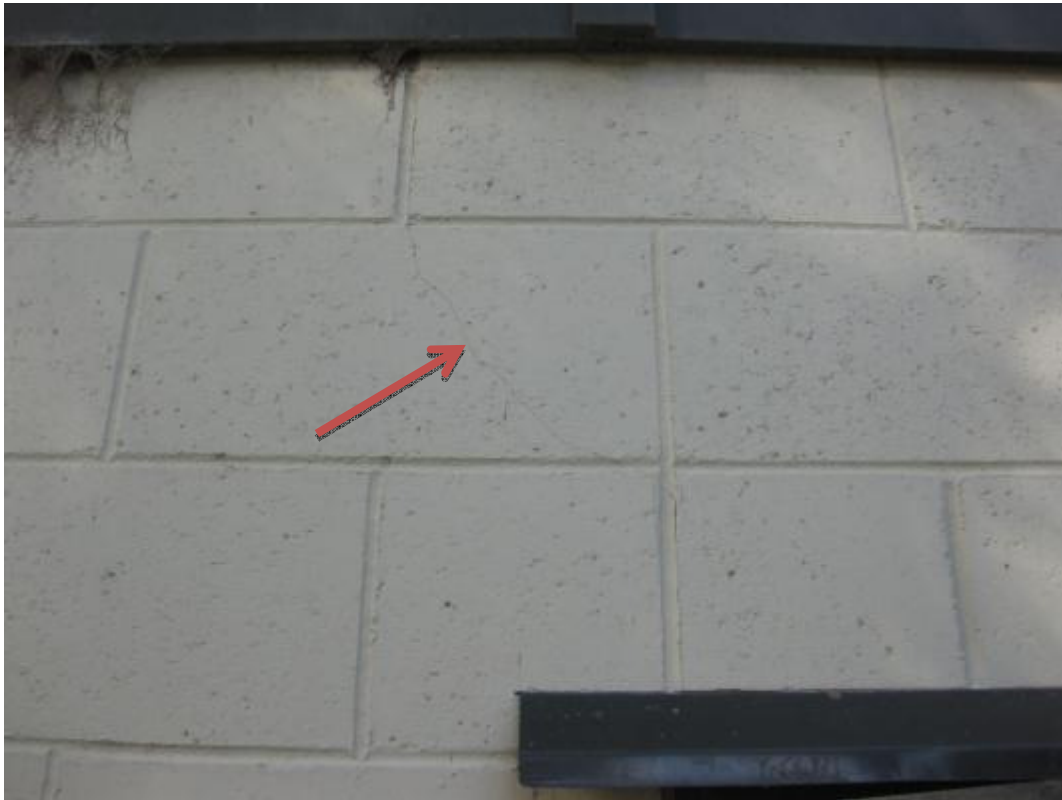
Photo 5: Crack in the south side wall above the door opening
