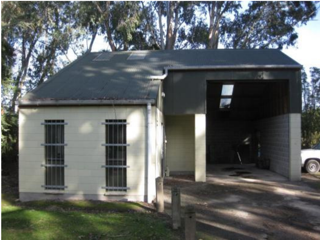
Photo 1: View of the building from north
