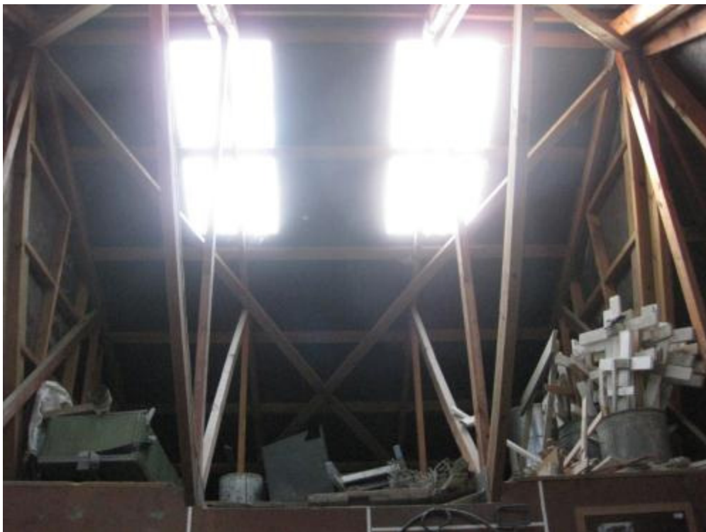
Photo 4: Roof frames and cross bracing of original building
