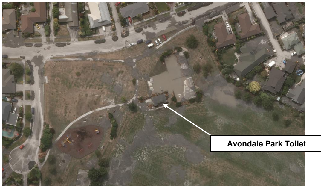
Figure 4 Post February 2011 Earthquake Aerial Photography
