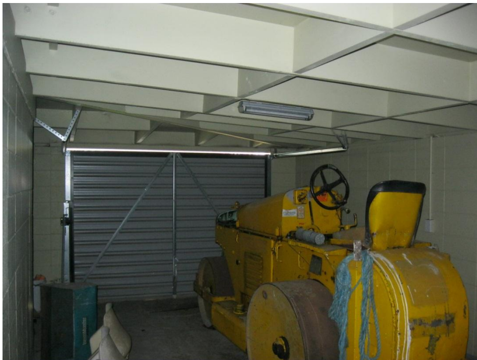
Photograph 6: Interior of the Storage Room
