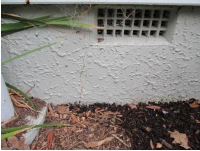
Minor cracking on perimeter concrete foundation
