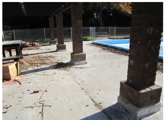
Photo 8: Four shelter support columns north of the building, spaced at 3.6m centres.
