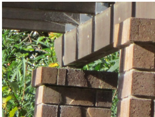
Photo 15: Timber elements on top of brick column.
