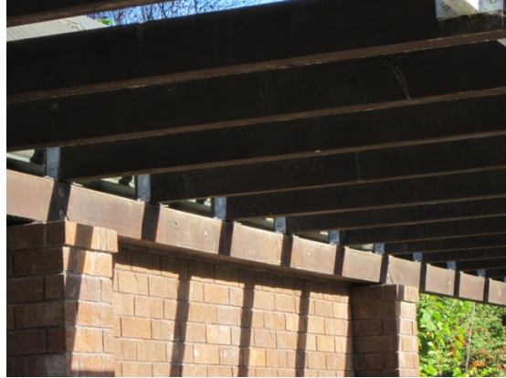
Photo 9: Timber beams in shelter.
