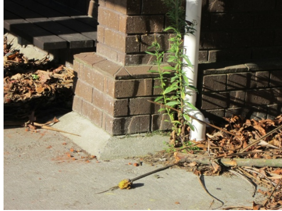
Photo 13: Base of brick column.
