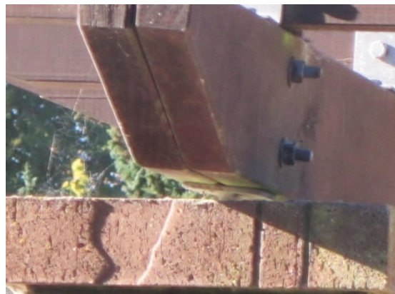
Photo 16: Timber rafter on top of brick column.
