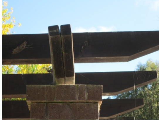
Photo 17: Warped timber element on top of brick column. Not believed to be earthquake damage.
