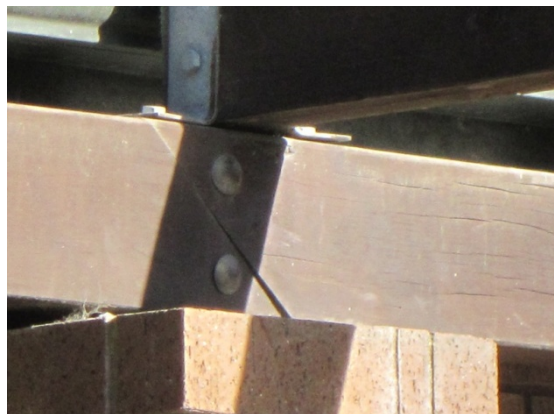
Photo 11: Connection in timber rafter on top of brick column.
