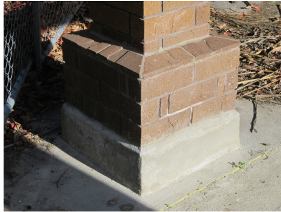
Photo 5: Base of brick column northeast of building.
