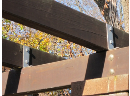
Photo 14: Timber elements and connection on top of brick column
