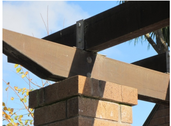
Photo 6: Top of brick column northeast of building. Connection shown between timber beams in the shelter.
