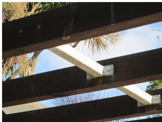
Photo 7: Steel hollow sections used as lateral supports between the timber beams of the shelter.
