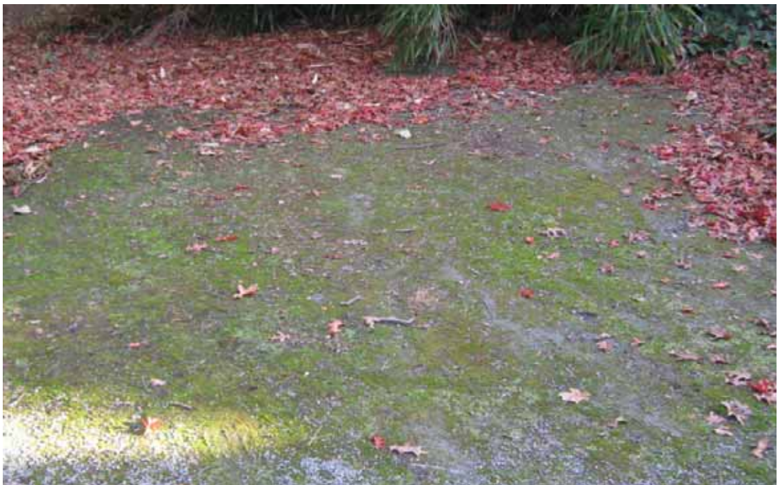
■ Figure 8 Evidence of sand and silt ejecta close by the toilet block and Pigeon Club buildings.
