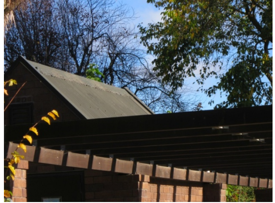
Photo 10: Timber beams in shelter.
