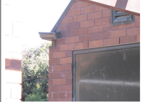
Photo 18: Dislodged gutter. Not believed to be earthquake damage.
