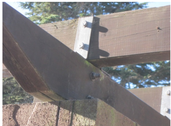
Photo 12: Timber elements and connection on top of brick column.
