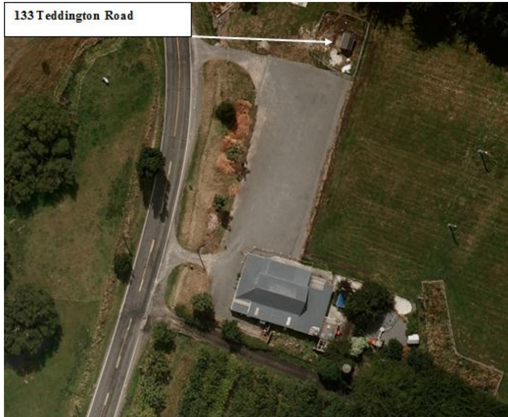
Figure 3 Post February 2011 Earthquake Aerial Photography 3
