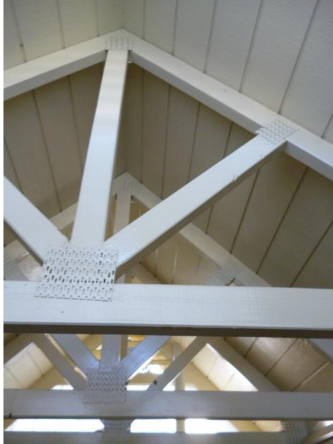
Photograph 5 Roof Trusses.
