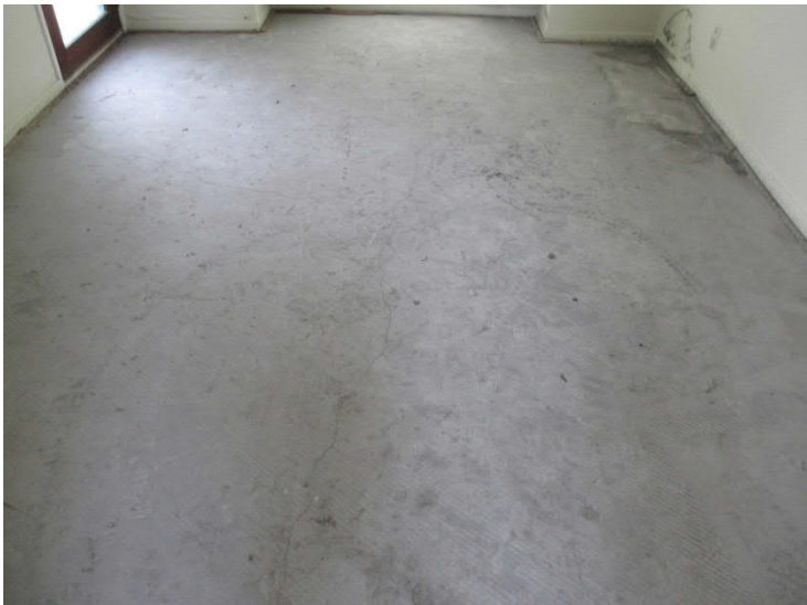
Cracks in the concrete floor (unit 2).
