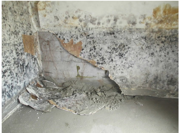
Liquefied silt inside the building. Silt has penetrated inside the timber walls (unit 4).
