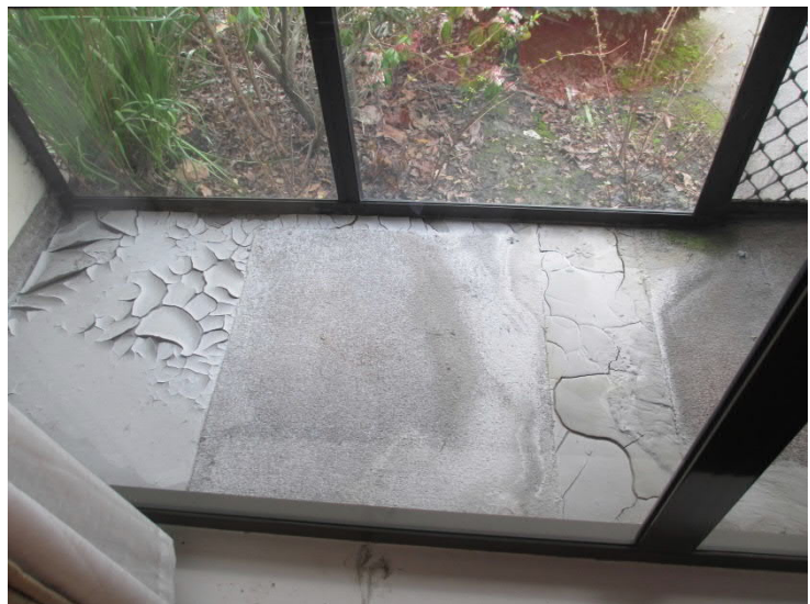
Liquefied silt inside the building (unit 2).
