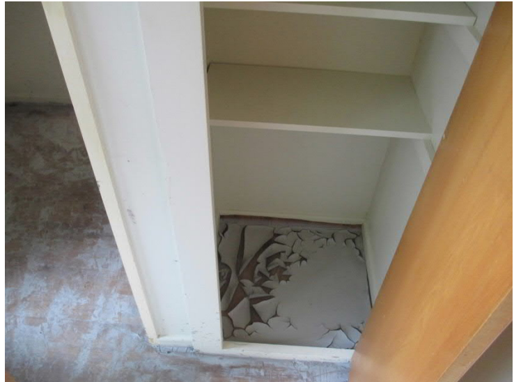
Liquefied silt inside the building (unit 2).
