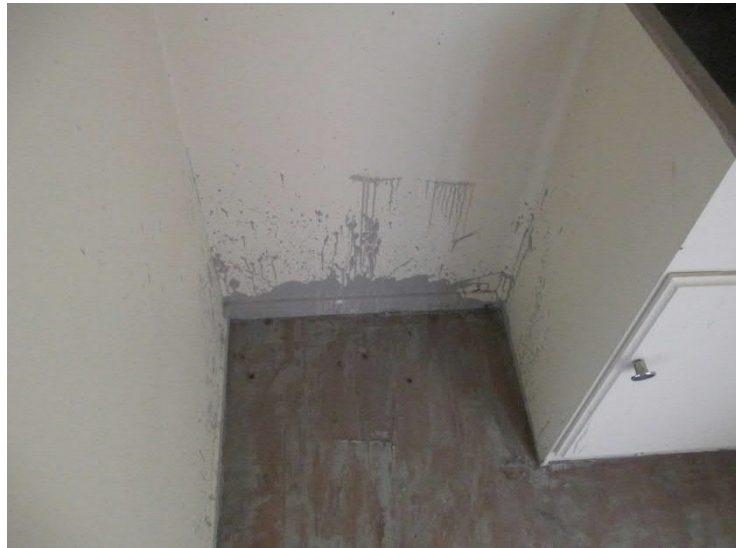
Liquefied silt inside the building (unit 2).
