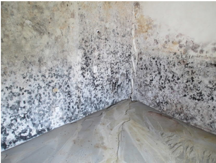
Liquefied silt inside the building (unit 4).
