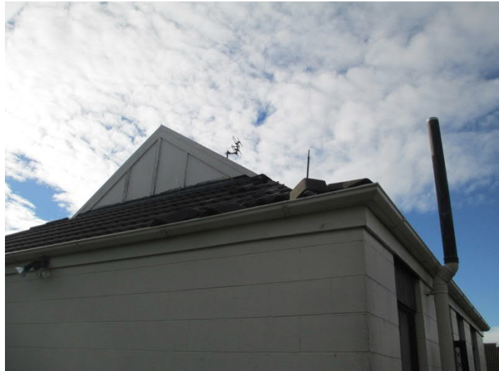
Movement of the roof tiles (unit 12).
