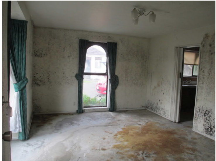
Liquefied silt inside the building (unit 4).
