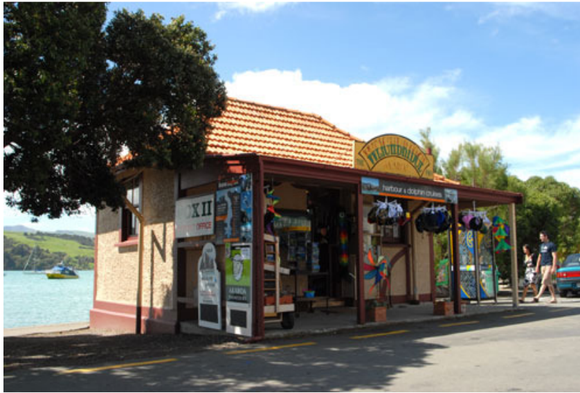
Figure 1: Akaroa Weighbridge Building
