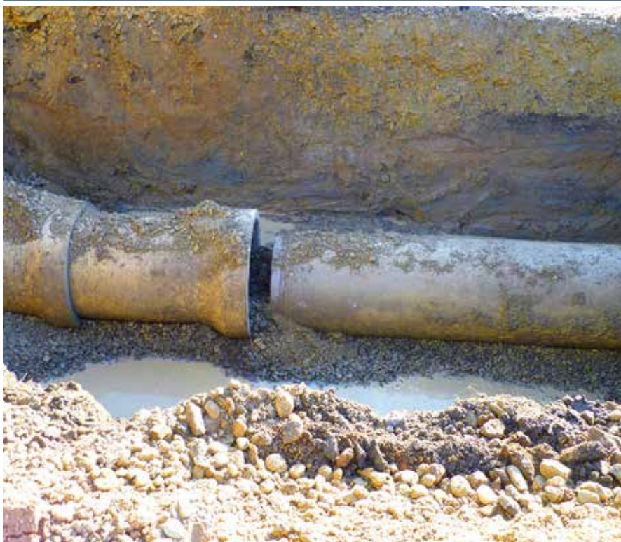
Earthquake damaged pipe
