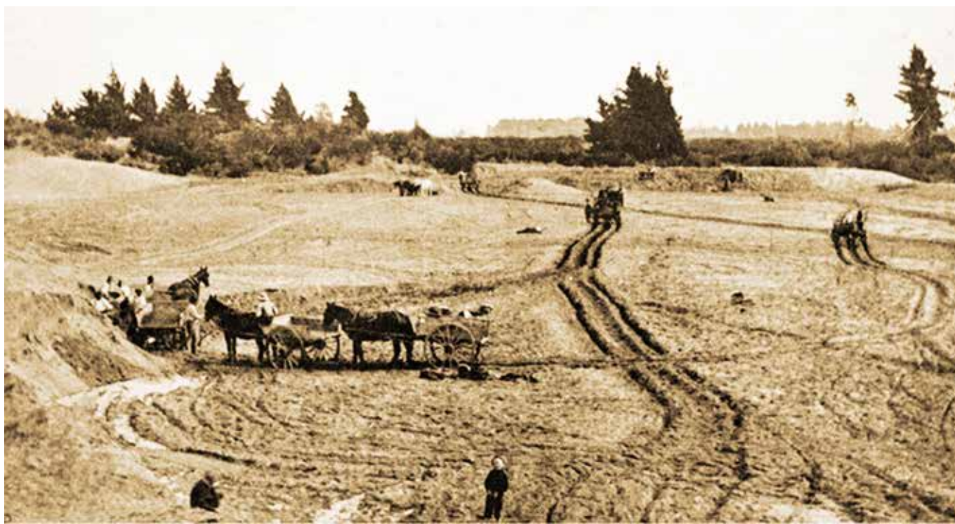
Levelling sandhills for Christchurch Drainage Board's Sewage Farm in Bromley 1904
