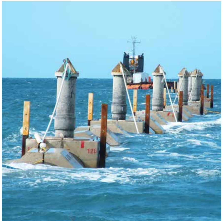
Ocean outfall pipe section on its way to seabed
