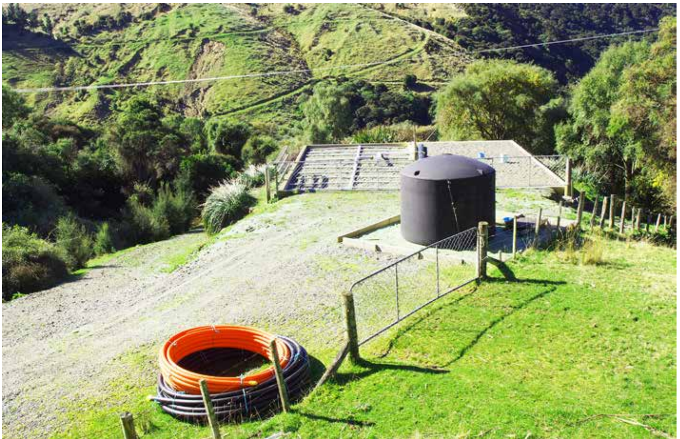
Wastewater treatment plant, Tikau Bay
