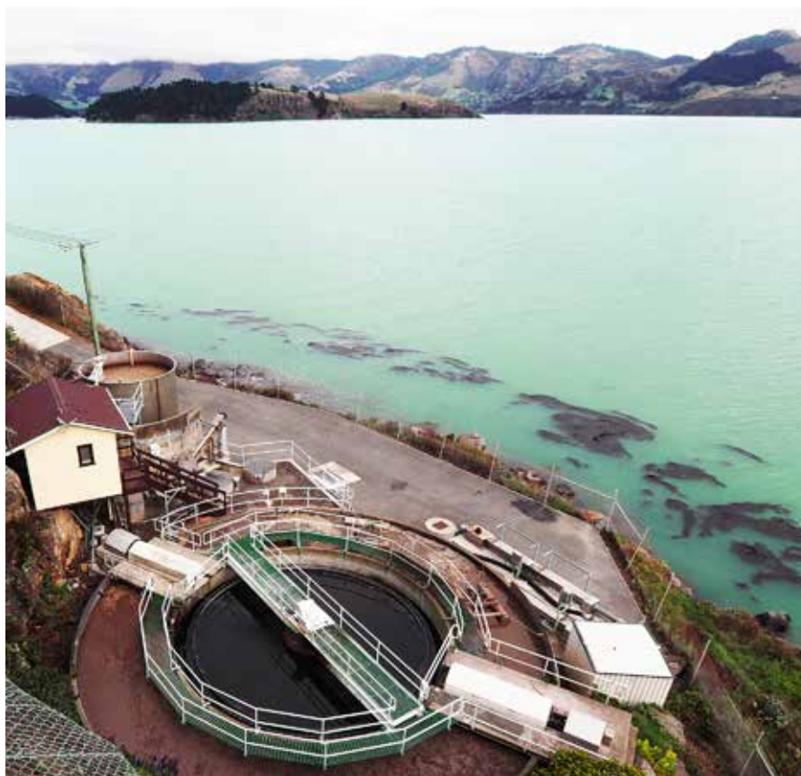
Wastewater treatment plant, Diamond Harbour
