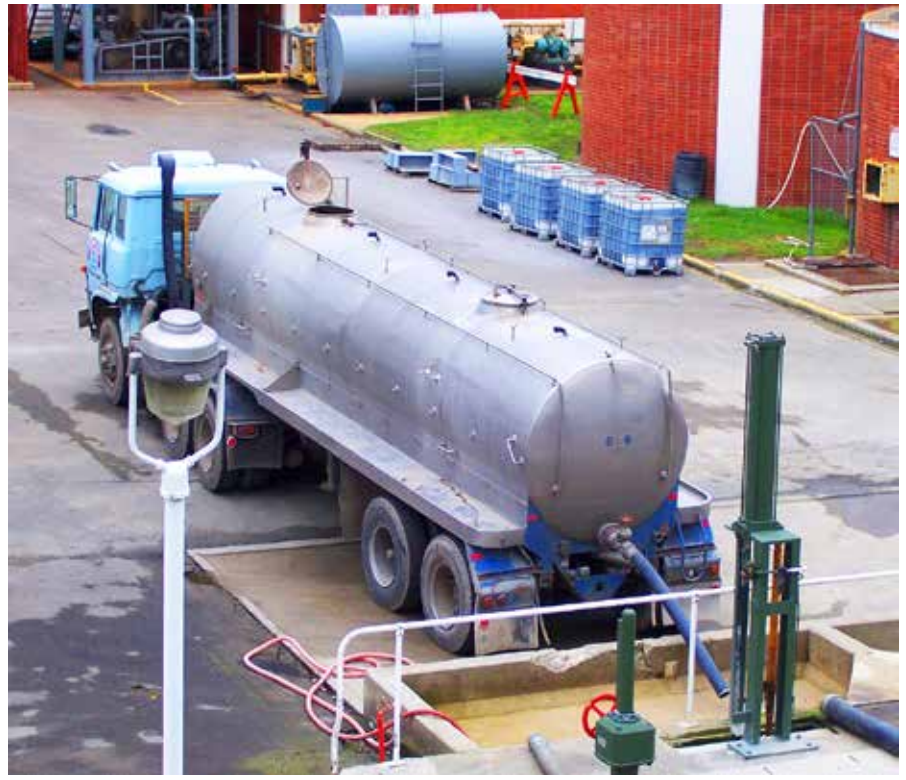
Tanker waste reception facility, Christchurch wastewater treatment plant
