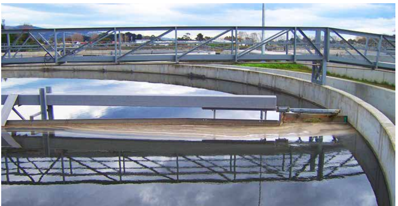
A clarifier at Christchurch wastewater treatment plant
