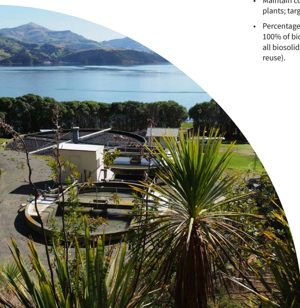
Akaroa wastewater treatment plant – Kelvin McMillan
