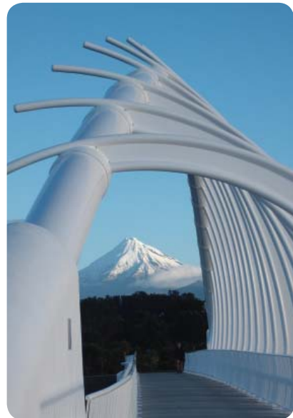
The Te Rewa Rewa bridge on the New Plymouth award winning coastal pathway.
