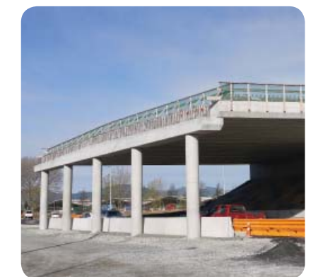
Construction of the Southern Motorway
