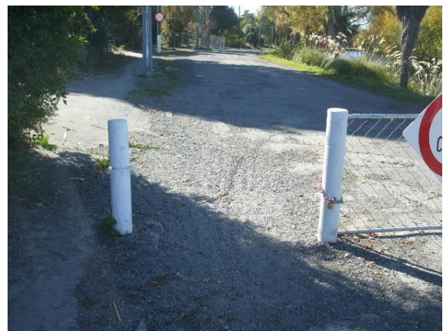
Figure 9: Existing road to be repaired and better signage
