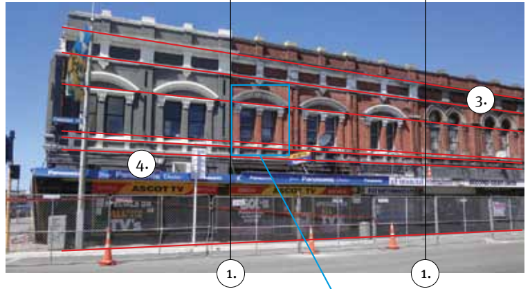
Demonstrating design elements on the Victorian Beverley Building
