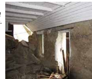
Figure 18: Original Penfolds Cottage (source: NZ Historic Places Trust), and earthquake damage to the cob cottage.
