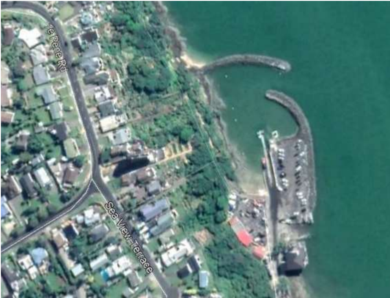
Maritai ramp, one within breakwater and one facing into open sea.
