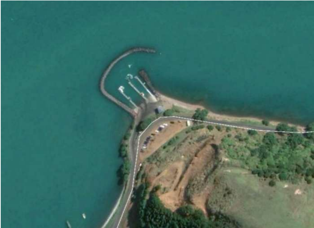
Kawakawa Bay club ramp, area open to wave action from north west through to north east.
