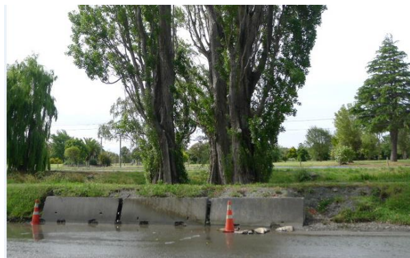
Figure 2: Example of trees within a section of stopbank on Avonside Drive to be removed (opposite Avon Park).
