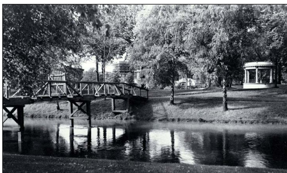
Figure 1.22. View of the Woodlands Bridge photographed between 1960 and 1972.
