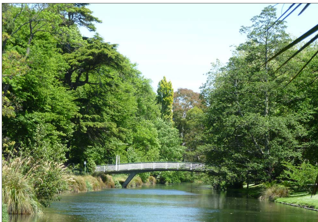
Figure 1.23. View of the Woodlands Bridge spanning the Avon River 2010.
