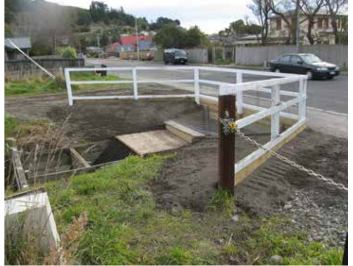
Completed Martindales Road culvert
