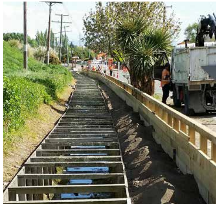
Work on culverts across Truscotts Road
