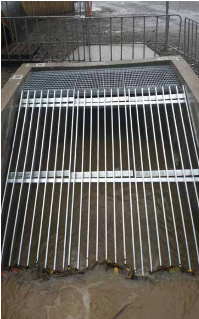
Bridle Path Stream intake under Port Hills Road
