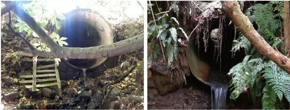
Figure 3: Church Lane Drain (Site 6, left) is a perched culvert assessed as presenting a very high risk to fish passage. The culvert on Wainui Valley Stream Branch (Site 9, right) likely presents a similar risk to fish passage, but the stream location was not mapped in the FPAT app, so a risk score was not calculated for the structure.
