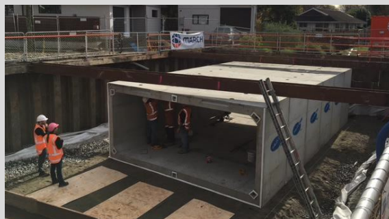
An example of a sheet piled trench on Warden Street. Note: The trench on Hills Road will be a lot smaller.
