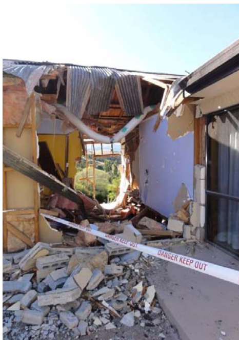
▲ Rockfall damage to a residential home at Rapaki Bay. This rockfall damage occurred in the main 22 February 2011 earthquake.
