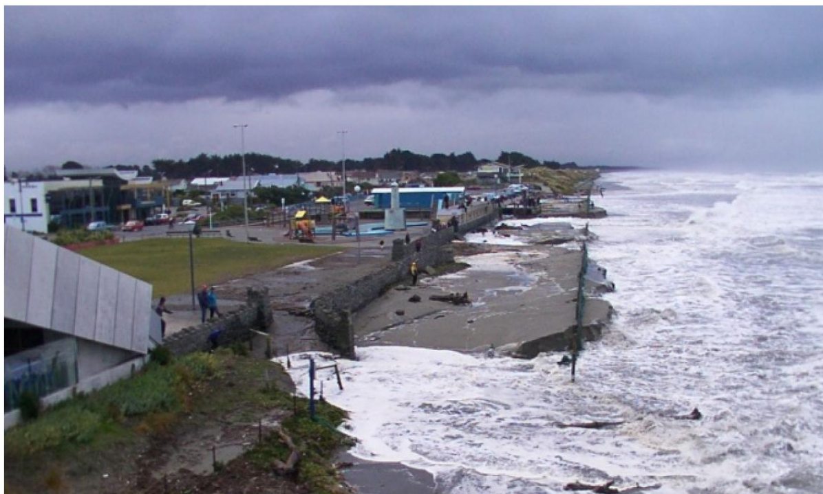
Figure 4-7: New Brighton pier area during the July 2001 storms (source: Justin Cope, ECan)
