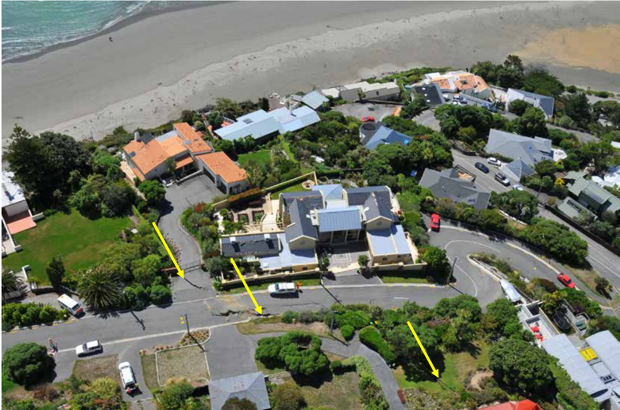
Figure 4 Tension cracks, shears and scarps (yellow arrows) formed by the 22 February 2011 earthquakes at the cliff crest cutting across Kinsey Terrace. Photograph G. Hancox (GNS Science, February 2011).
