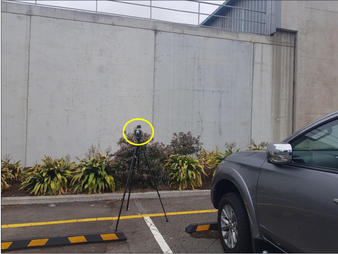
Figure 5. Living Earth Carpark, 18 December 2020.
