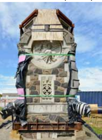
Temporary protection of the clock tower
