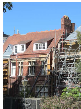
Temporary protection measures
