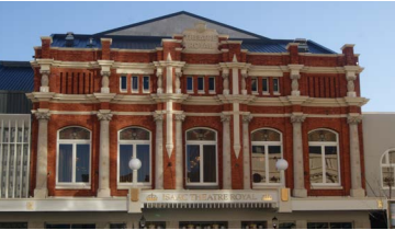
Repaired Isaac Theatre Royal Building
