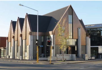
Repaired Knox Church exterior
