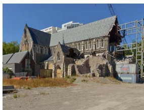
Earthquake damaged church, made secure
