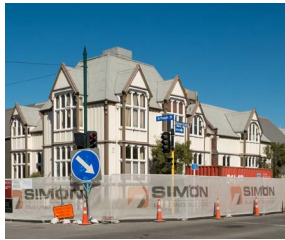
Temporary protection measures
