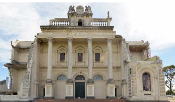
Earthquake damaged church, made secure
