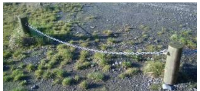
Gate Type = Vehicular Gate Style = Post and Cable Construction Material = Chain Post Material = Wood Surface Finish = Galvanised
