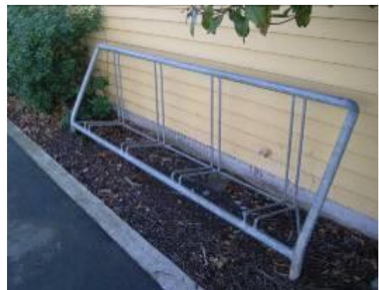
Steel cycle stand. Galvanised surface finish.
