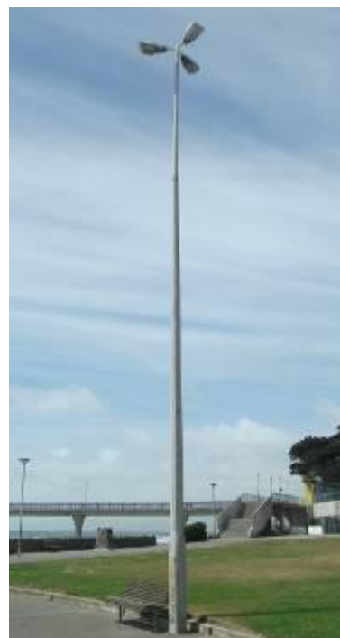
Concrete light pole with three floodlights. This pole has no surface finish.
