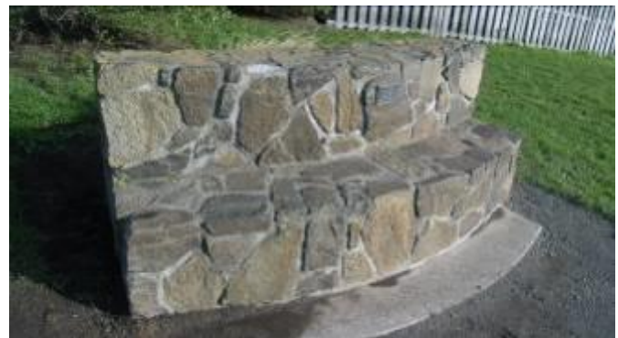
Stone seat fixed to the ground with a concrete footpad.
