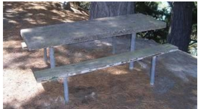
Picnic table with a concrete table top and steel frame. This table has no surface finish or footpad.
