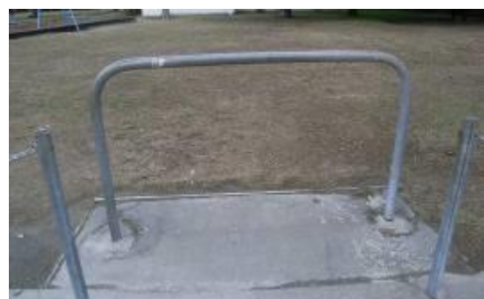
Steel Cycle Barrier, galvanised.
