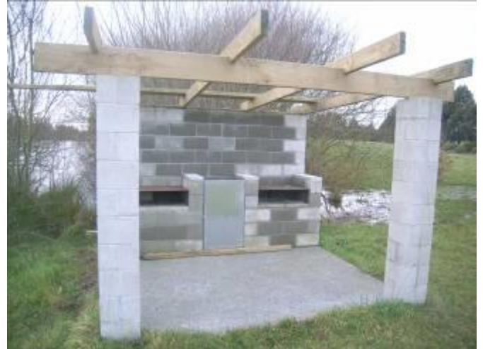
Open fire concrete block BBQ in a shelter.
