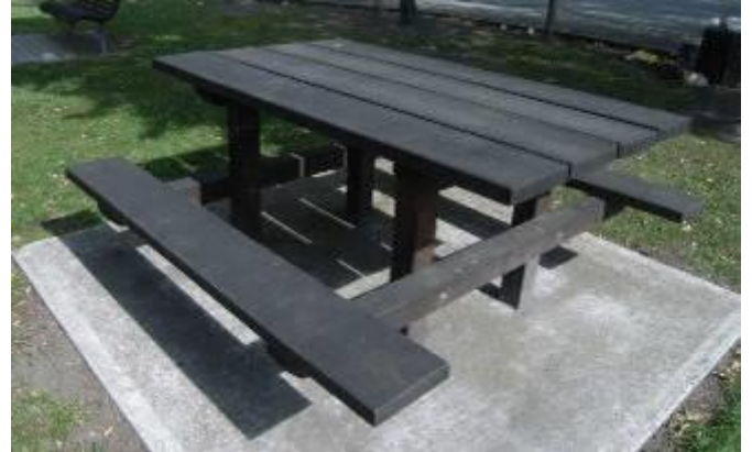
Picnic table with a wooden table top and frame, painted surface finish and concrete footpad.
