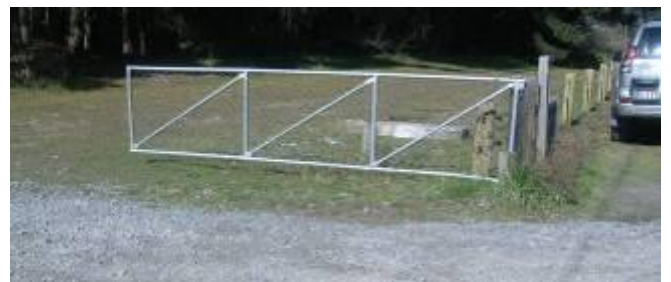
Gate Type = Vehicular Gate Style = Standard Farm Gate Construction Material = Steel Post Material = Wood Surface Finish = Galvanised
