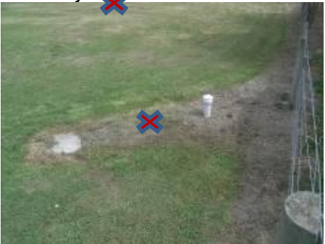
Buried Septic tank. Vent and access exposed.
