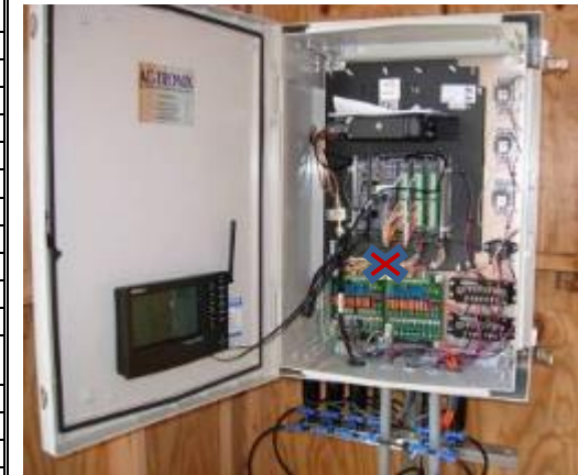
Irrinet system in wall cabinet.
