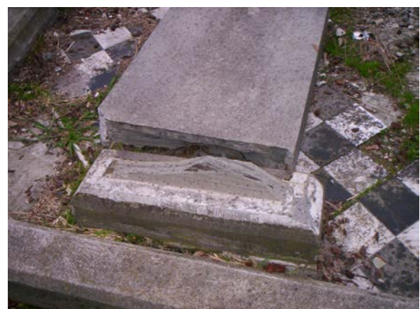
Slate headstone with a concrete skin
