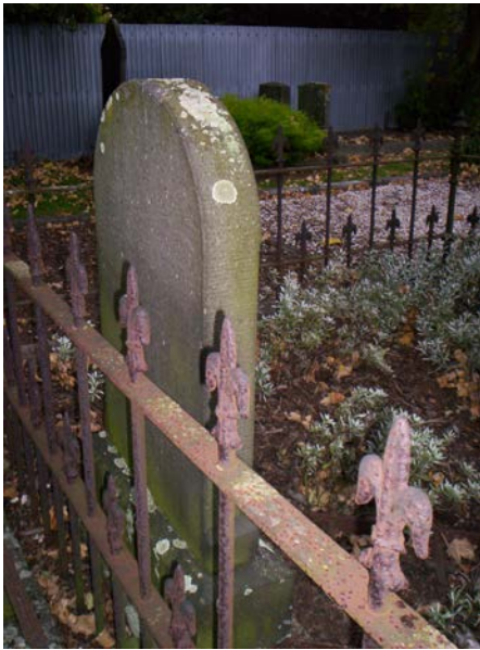
Headstone showing toolmarks on side and back, and iron railing with the common fleur-de-lys motifs
